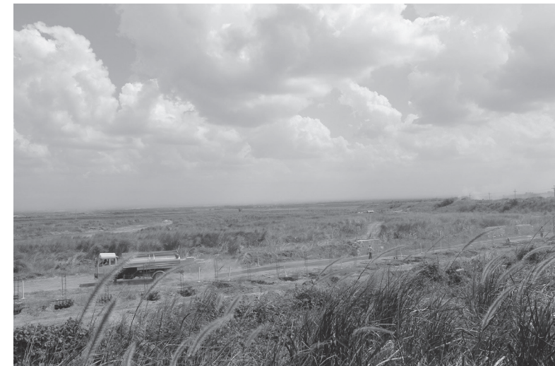
Fig.2. Ongoing Construction of Alviera as of February 2016
