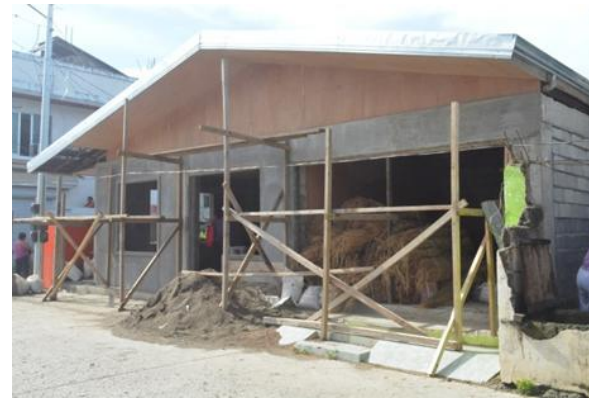
Construction of the new showroom after Typhoon Yolanda
