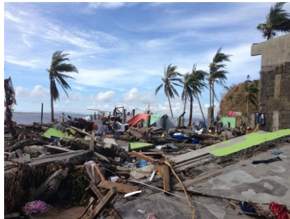
The storm surge has reached the showroom of Eva Marie Arts and Crafts Inc. and completely destroyed the building and the products inside.
