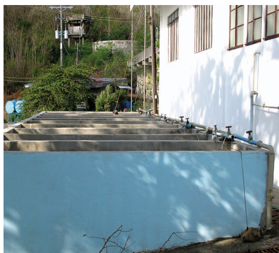
Concrete tanks for tilapia culture at SEAFDEC/AQD, Binangonan Freshwater station, Rizal, Philippines. Photo by J.A. Ragaza.
