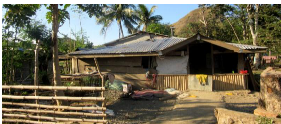
Figure 5. Typical house with a 30 W solar PV system.
