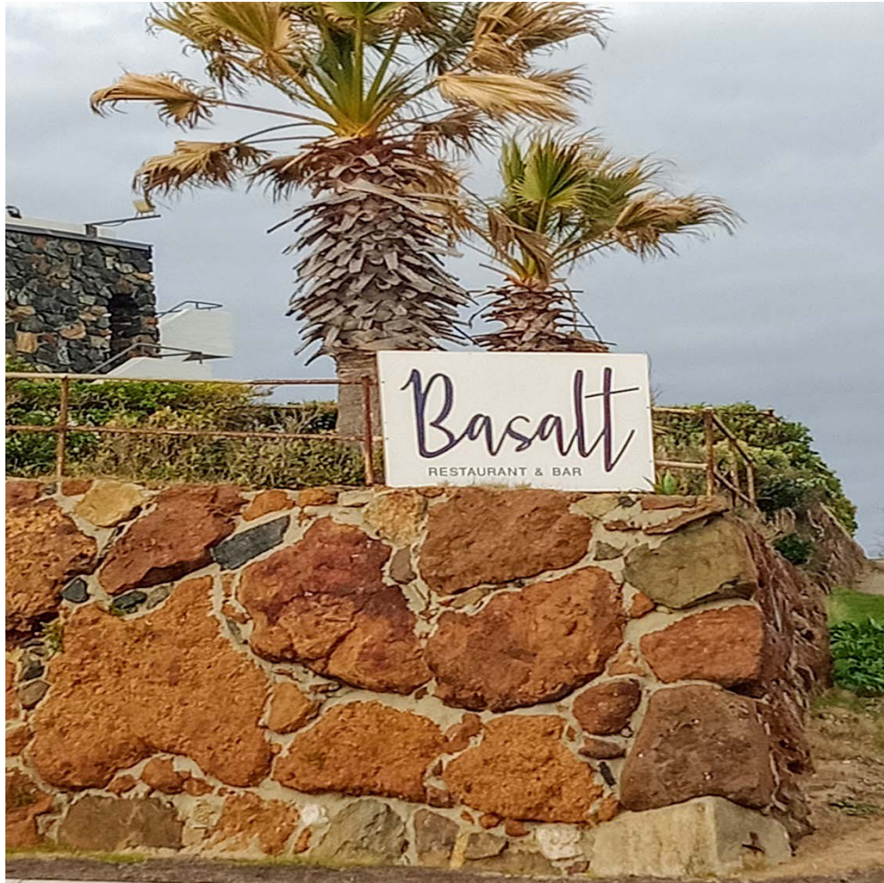
Figure 4.2.1. The Lighthouse Hotel, featuring the rubblestone masonry and Ferruginous duricrust of its retaining wall (foreground), ashlar stonework (top left) and arched window frame, reflecting 18 th and 19 th -century rustication techniques. Photograph by S. Richards.
