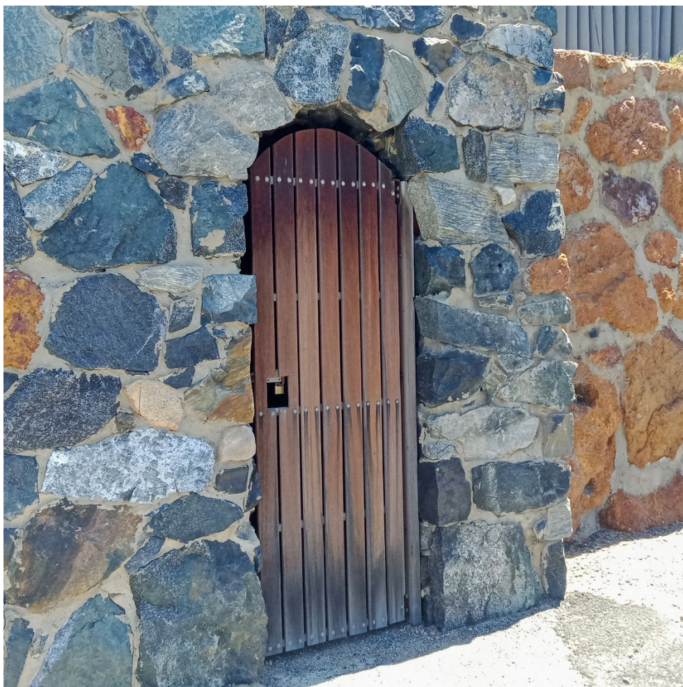
Figure 4.2.2 Richardson Romanesque style arched doorway featuring ashlar (finely cut) stonework and rubblestone (uncut stone) wall (right) of the Lighthouse Hotel. Photograph by S. Richards.
