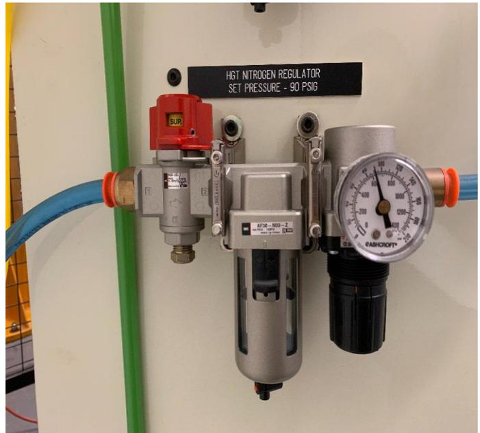
Figure 22. Nitrogen supply line (Left); HGT nitrogen regulator (Right)
