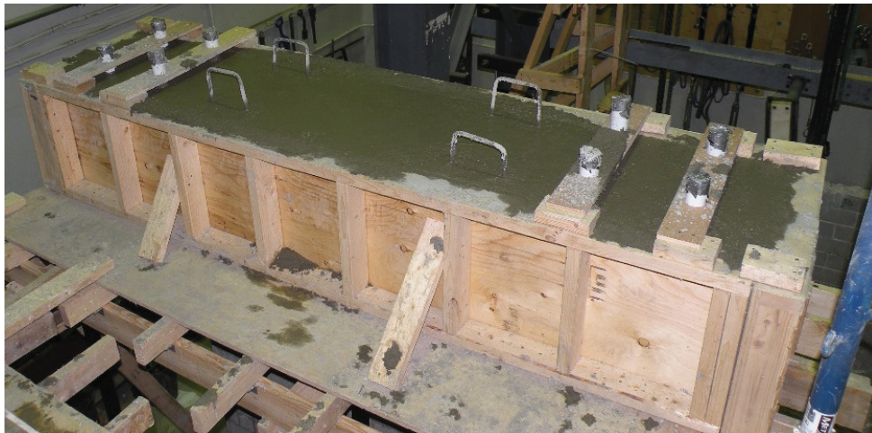
Figure A.5 Top footings' formwork, reinforcement and concrete
