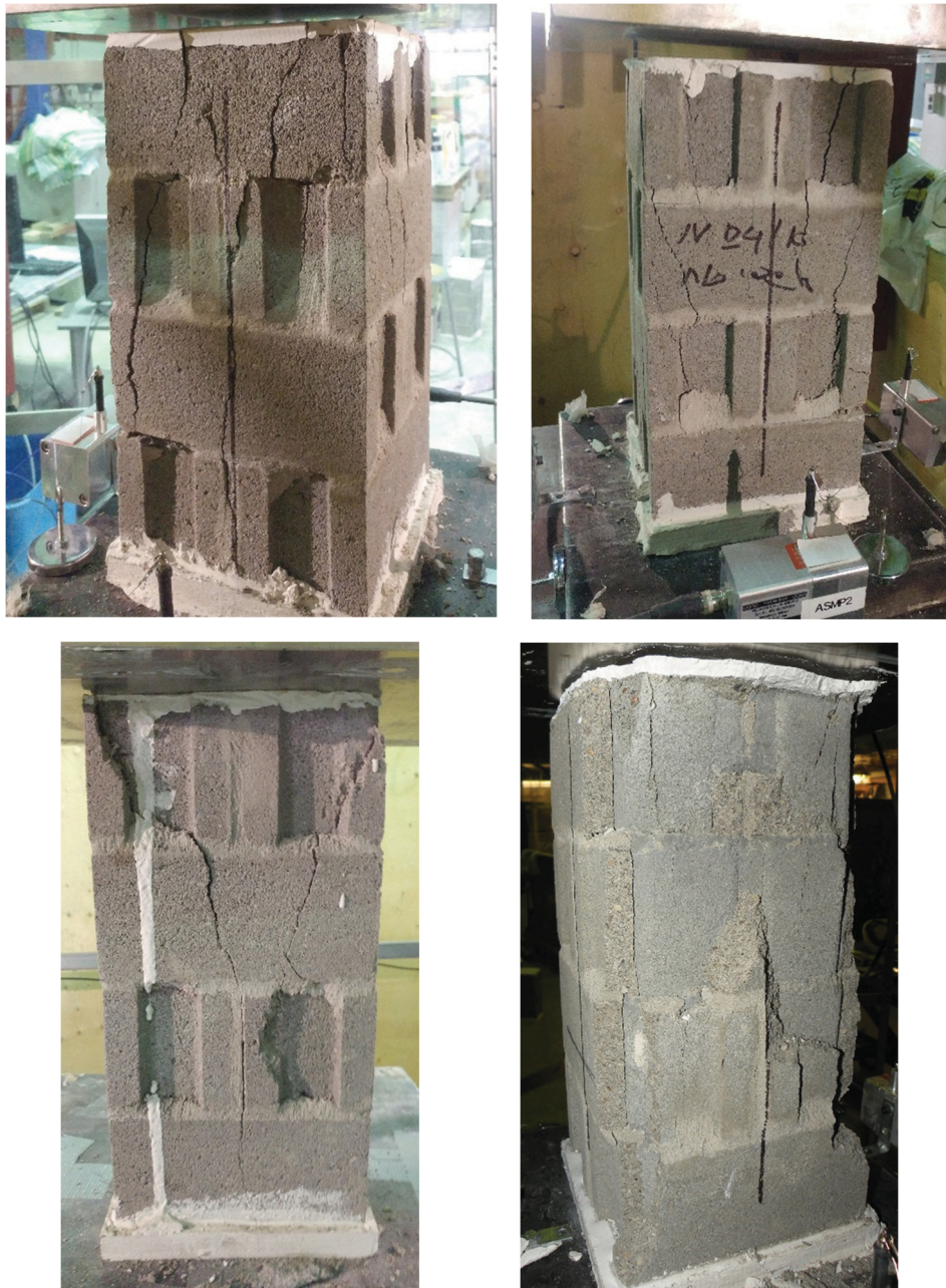
Figure A.28 Typical final damage states of tested boundary element (stretcher blocks) prisms
