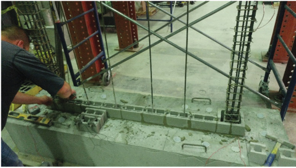
(1) Laying 1 st masonry course
