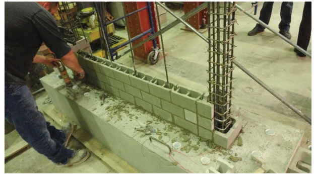
(2) Laying 2 nd & 3 rd masonry course
