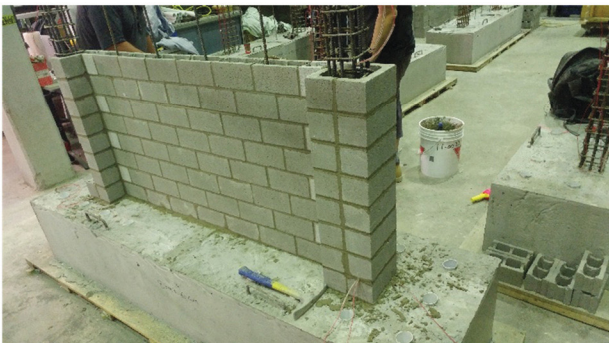
(5) Completing 1/3 of the wall height
