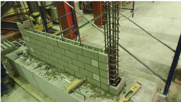
(3) Laying 4 th & 5 th masonry course
