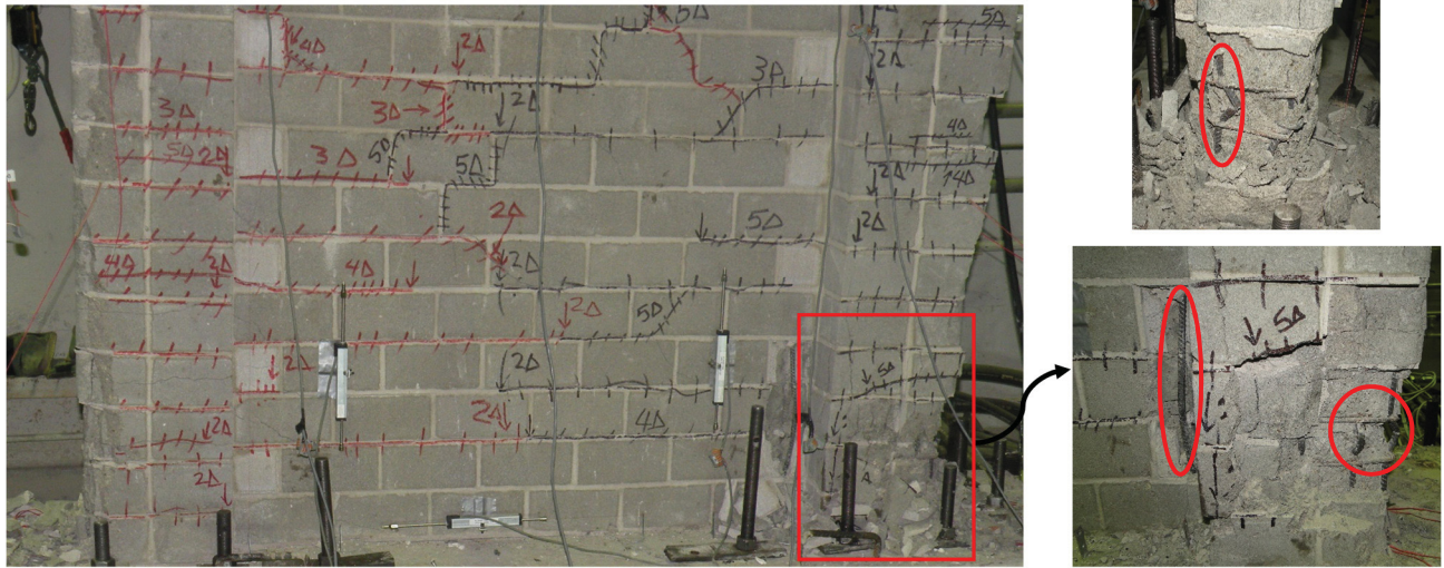
Figure A.8 Final damage state and failure of wall W9
