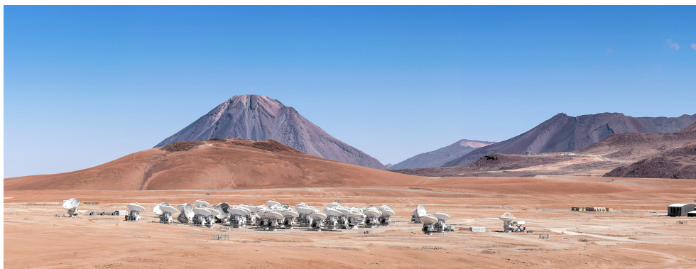
Figure 1.10: 66 ALMA antennas installed in a clear compact configuration. In the background is the Licancabur Volcano and on the far right is Chajnantor hill. Credit: ALMA (ESO/NAOJ/NRAO)
