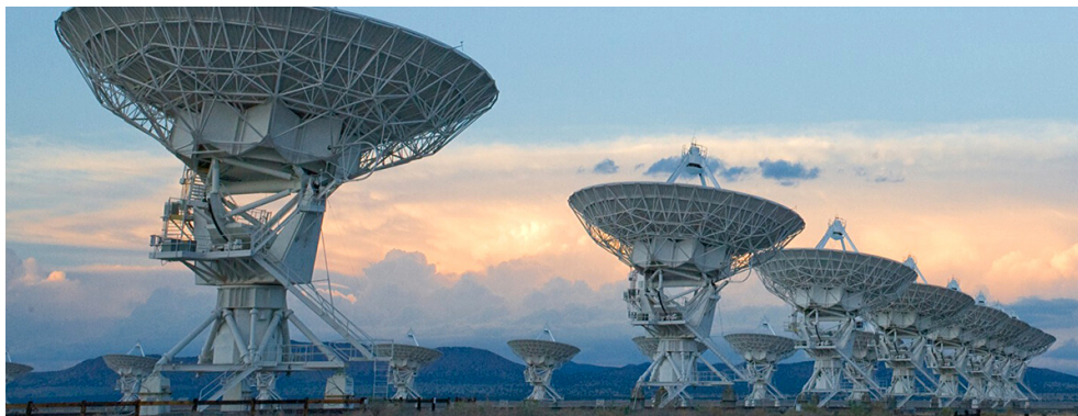
Figure 1.9: The Very Large Array (VLA) is a collection of 27 radio antennas located at the NRAO site in Socorro, New Mexico. Credit: Alex Savello.
