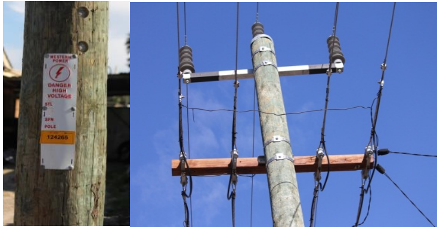
Figure 3-10. Replaced wooden power pole
