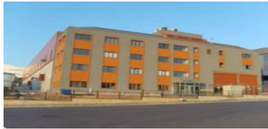
Figure 4-2: General view of the subject plant
