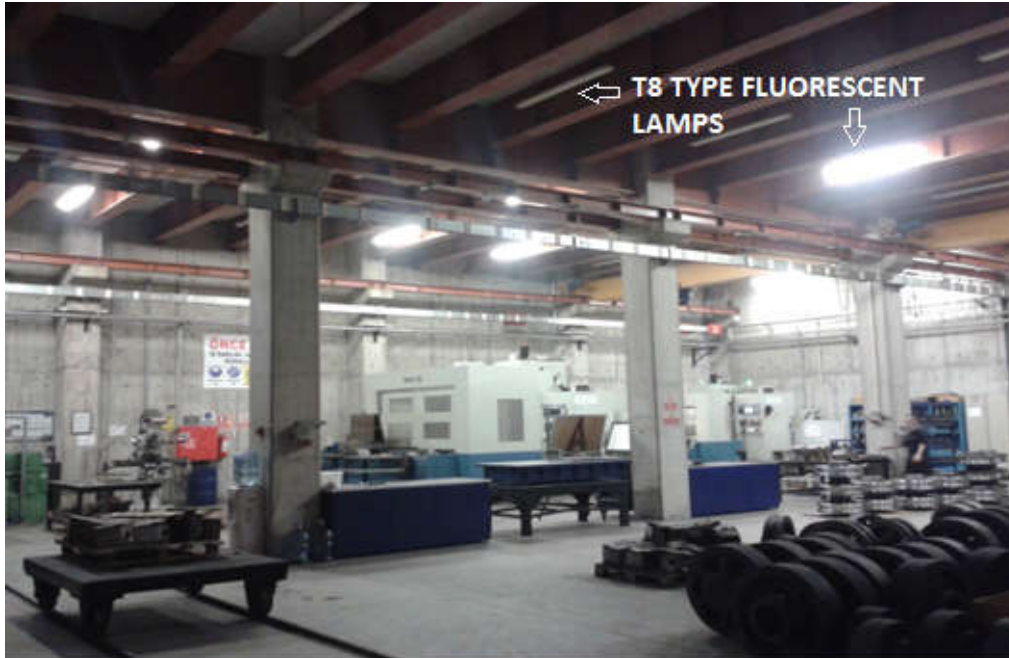
Figure 6-65: Machine shop in the basement floor of the subject plant
