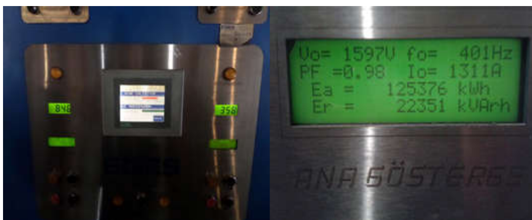
Figure 5-2: Melting Furnaces Power Meter and Control Unit in the Subject Plant (Photo taken by the Author)
