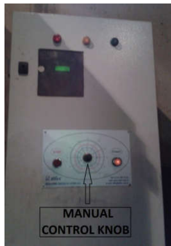
Figure 6-6: VFD used in the ventilation system (Photo taken by the Author)
