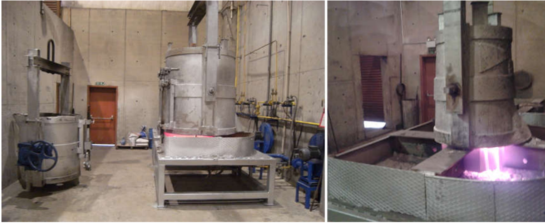
Figure 5-10: Ladle preheating in the subject plant (Photo taken by the Author)
