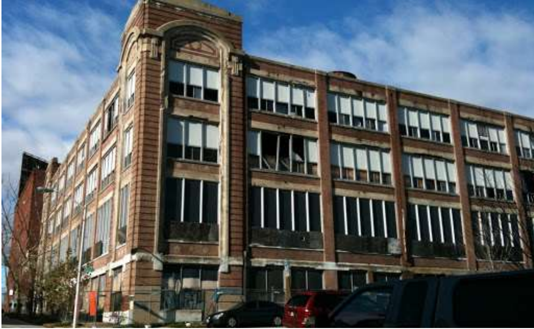
Figure 4.5. The former garment factory of 1500 Barclay sat vacant for decades with its features deteriorating. (Ziger/Snead Architects, 2010)
