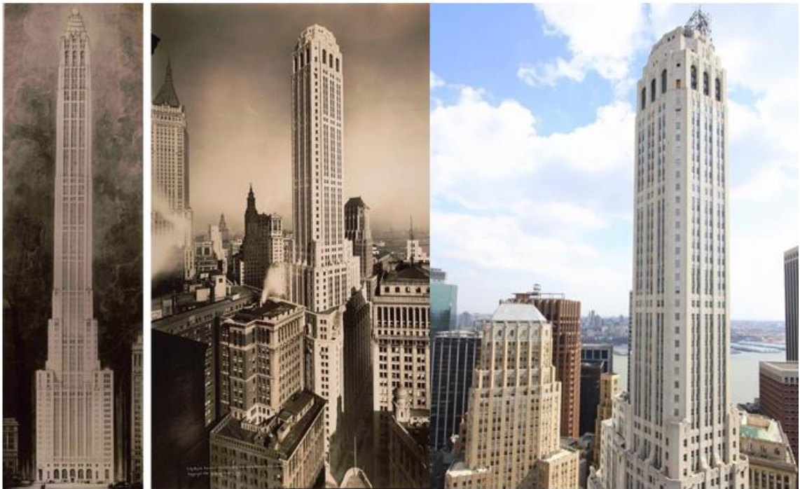
Figure 16. 20 Exchange Place, historic and current views. Picture made by the Author based on NYC Urbanism (Left: Original rendering from Cross & Cross. Middle: Twenty Exchange as built, 1931) & cityrealty.com (Right)
