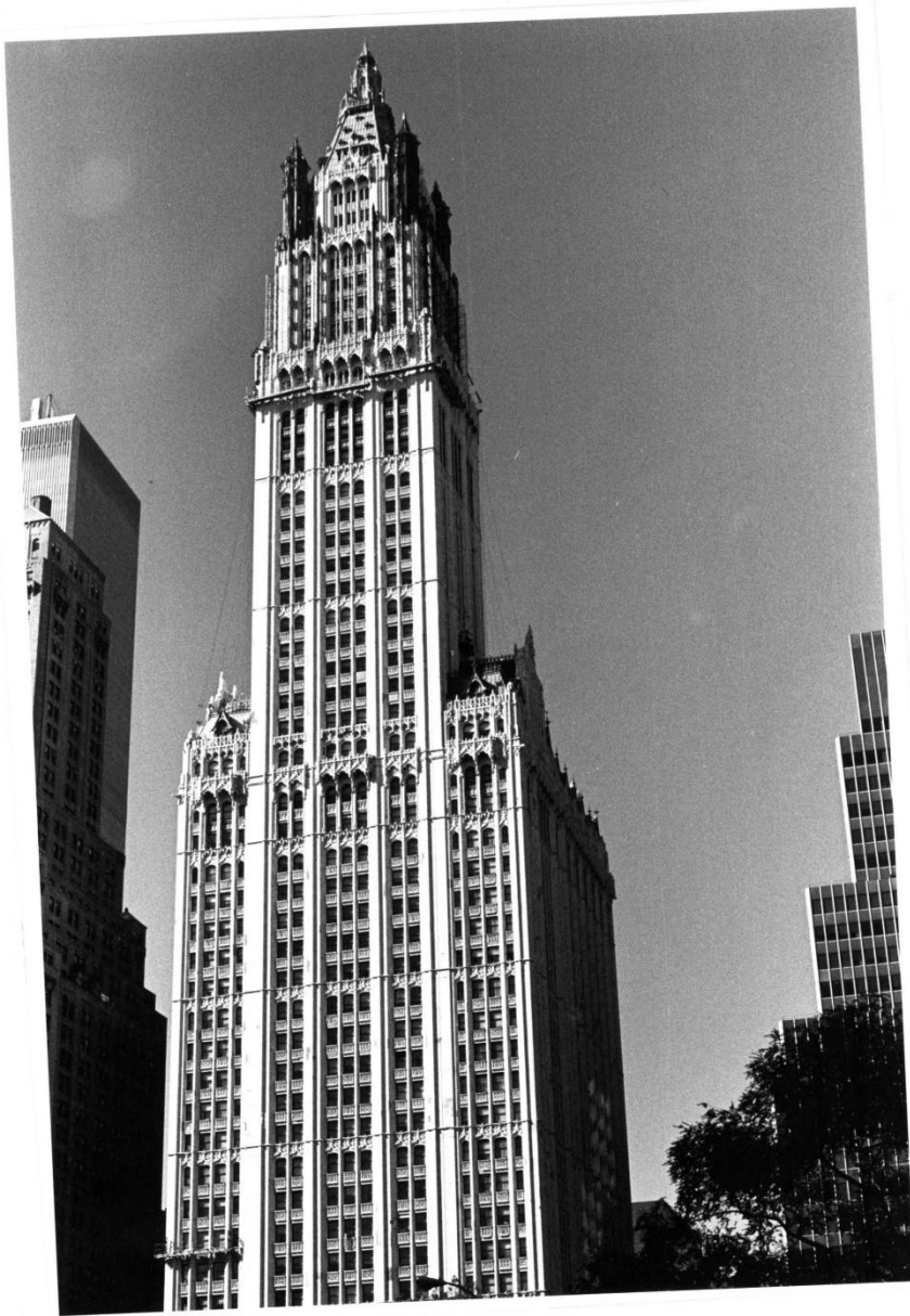
Woolworth Building 233 Broadway Manhattan
