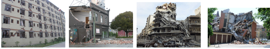
a (a) Original building-damage images
