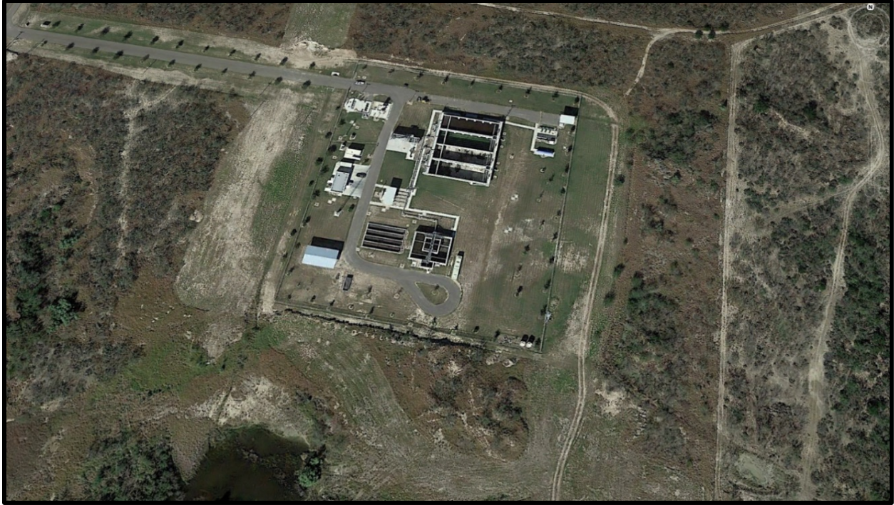
Figure 1-27. AGUA Special Utility District's Wastewater Treatment Facility.
