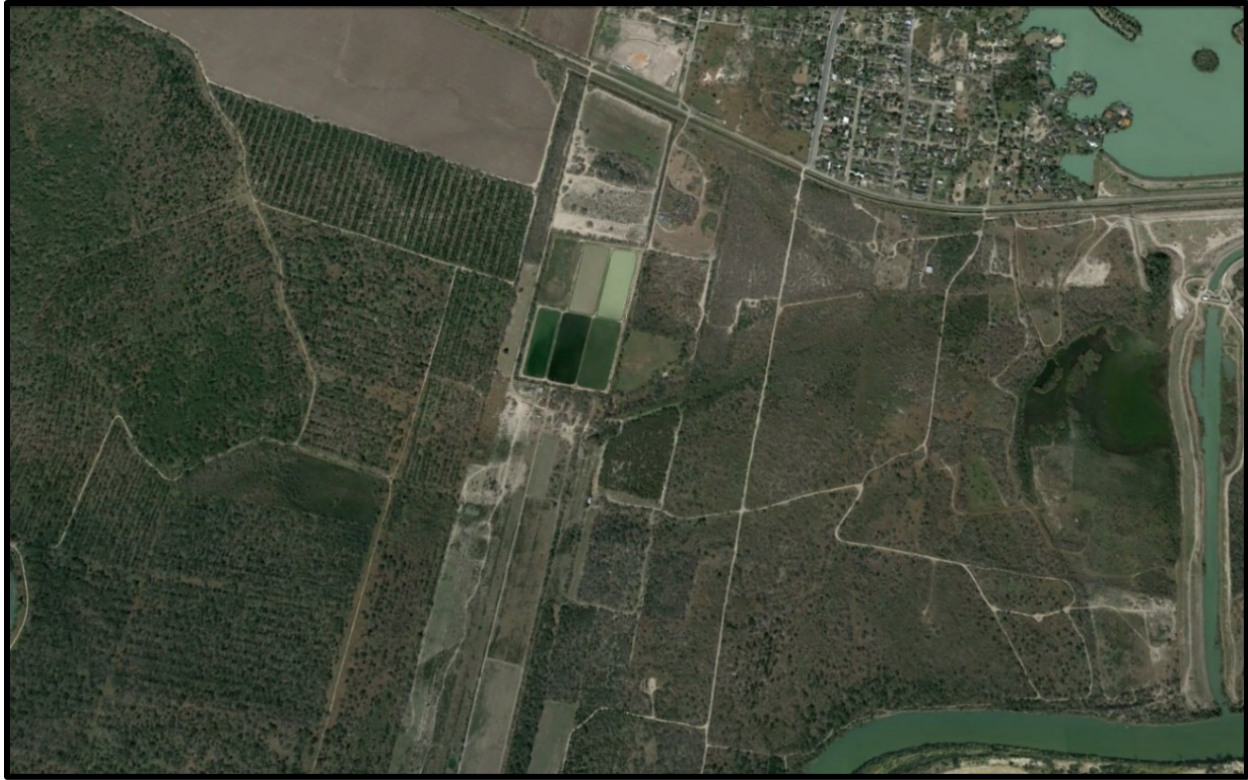
Figure 1-29. The City of La Joya's Wastewater Treatment Facility.
