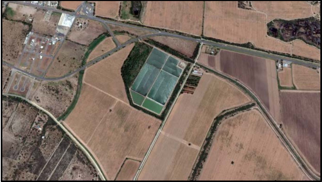
Figure 1-36. Ciudad Miguel Alemán's Wastewater Treatment Facility.
