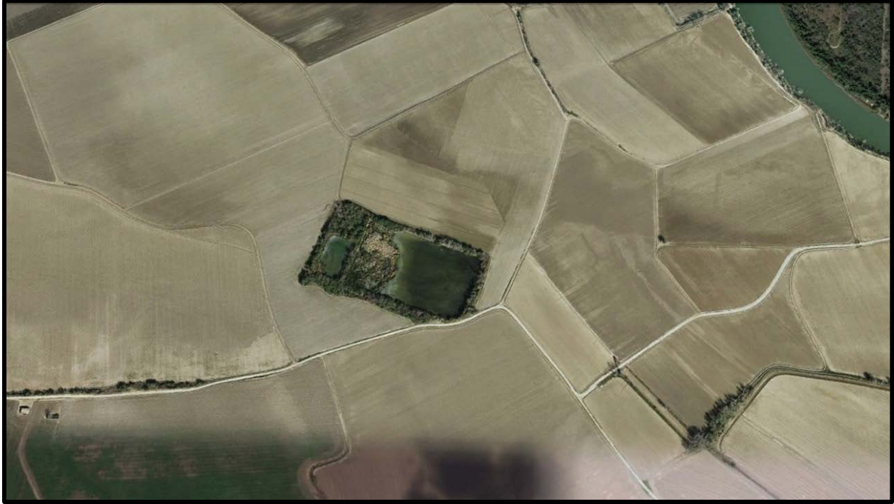
Figure 1-38. Ciudad Gustavo Díaz Ordaz's Wastewater Treatment Facility.
