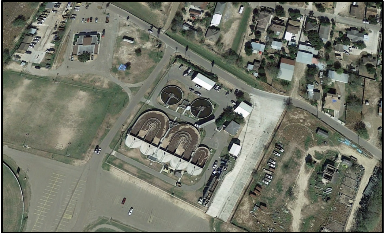
Figure 1-24. The City of Roma's Wastewater Treatment Facility.
