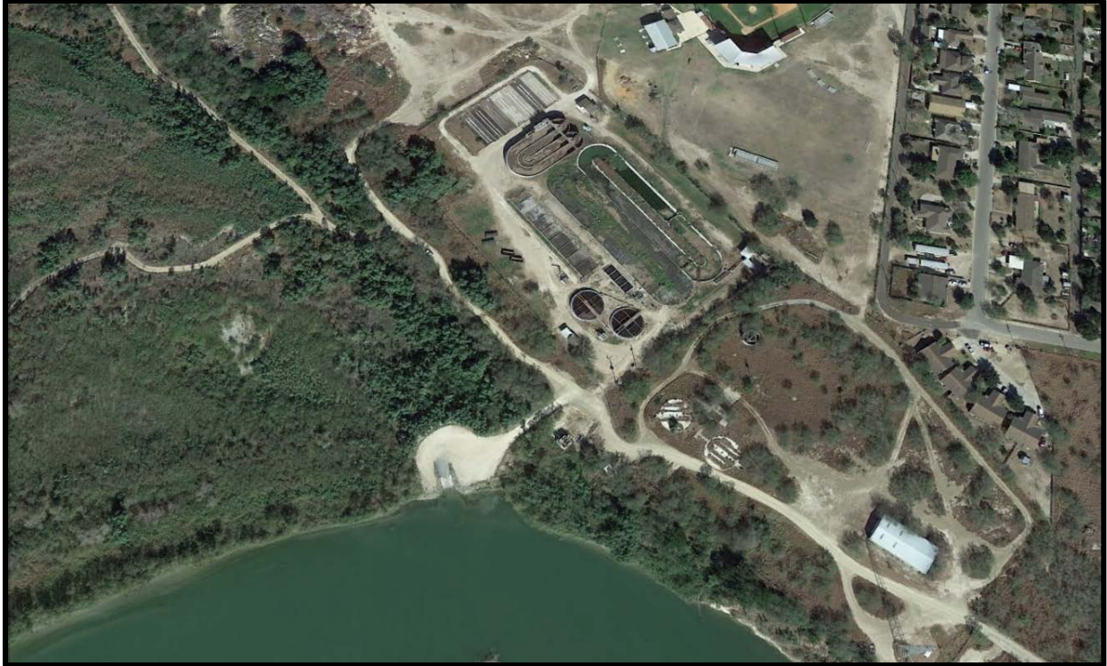
Figure 1-25. The City of Rio Grande City's Wastewater Treatment Facility.
