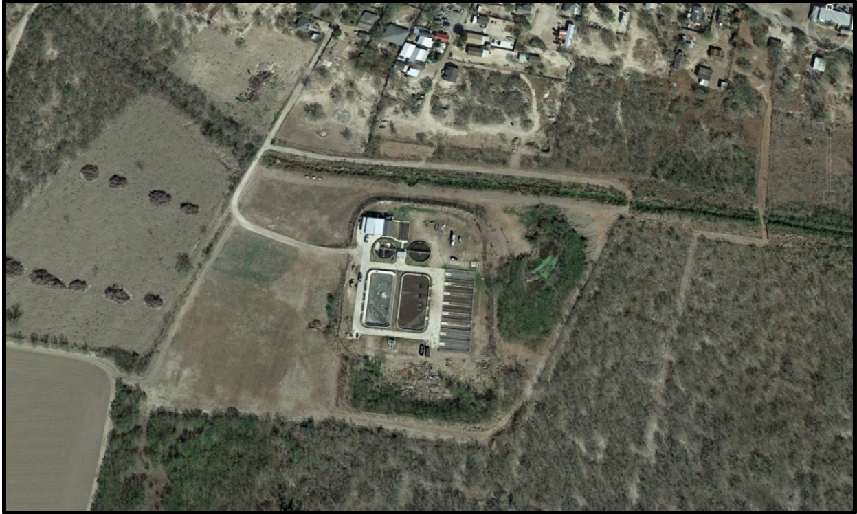
Figure 1-26. Union Water Supply Corporation's Wastewater Treatment Facility.
