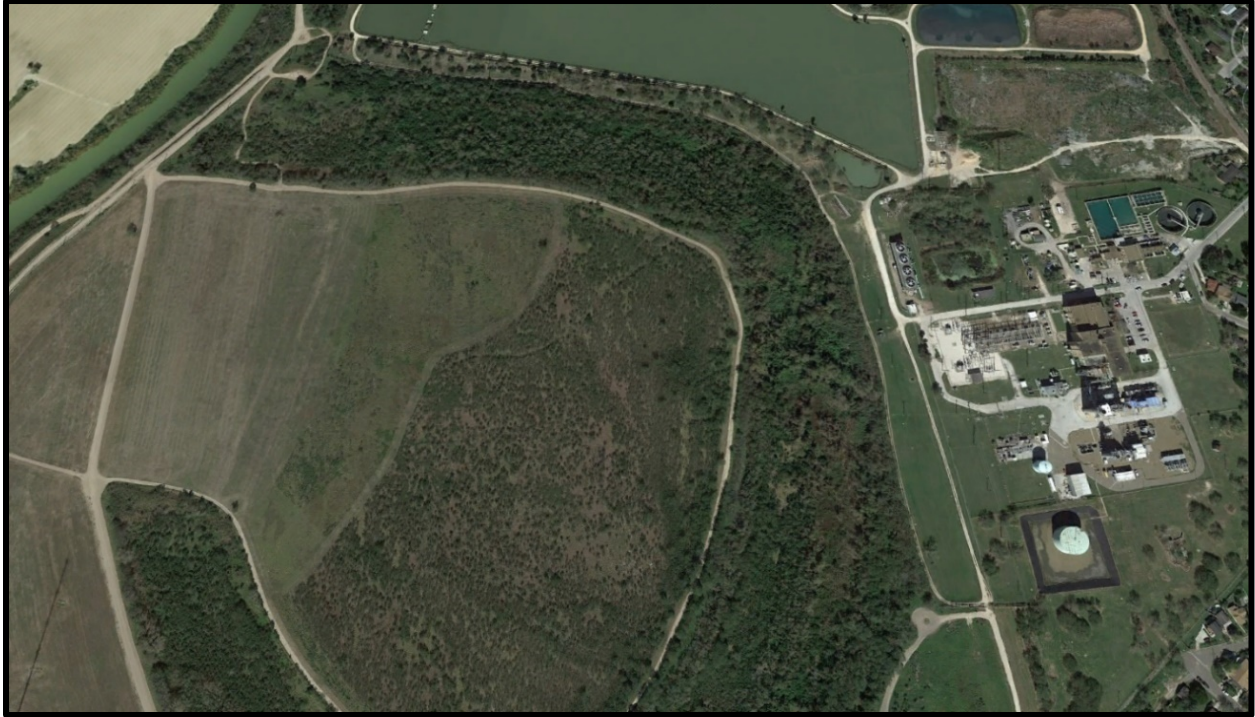
Figure 1-31. Brownsville Public Utility Board's (BPUB's) Silas Ray Power Plant.
