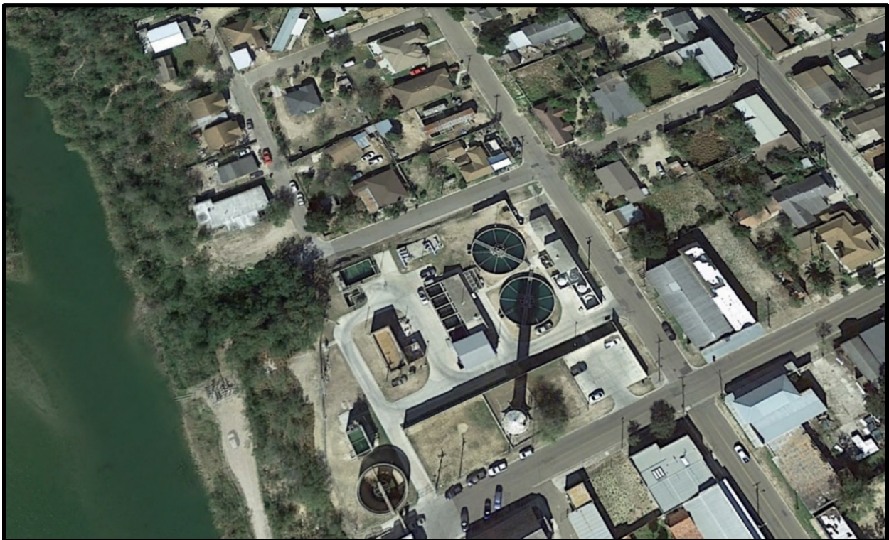
Figure 1-23. The City of Roma's Drinking Water Treatment Facility.
