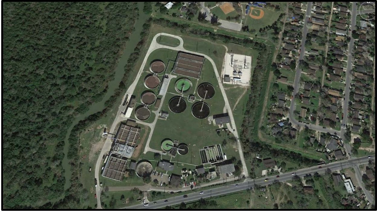
Figure 1-32. BPUB's South Side Wastewater Treatment Facility.
