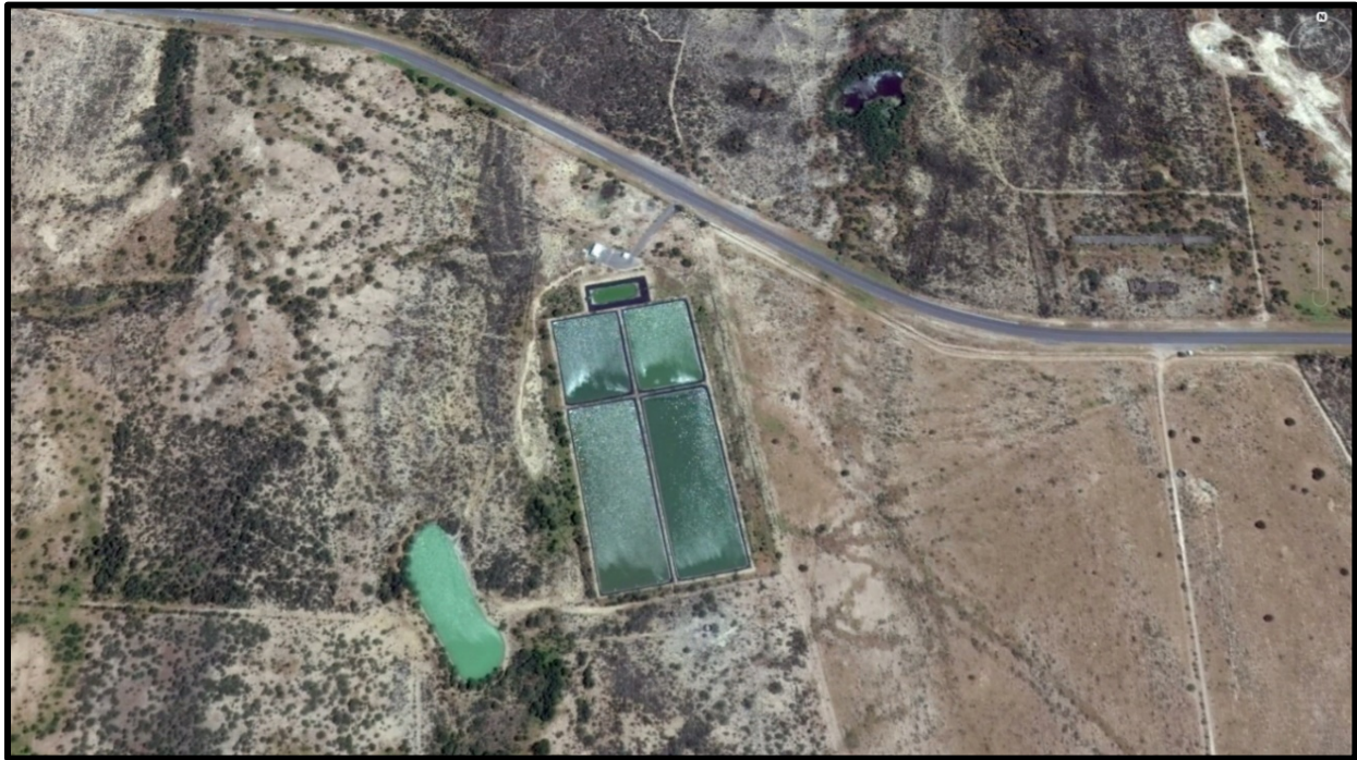
Figure 1-35. Ciudad Mier's Wastewater Treatment Facility.
