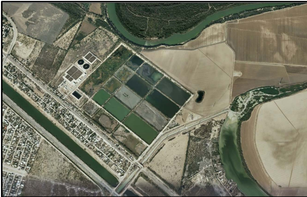
Figure 1-40. Ciudad Reynosa's Wastewater Treatment Facility No. 1 (PTAR No. 1).
