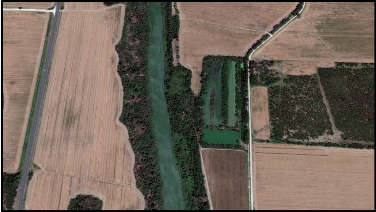
Figure 1-37. Ciudad Camargo's Wastewater Treatment Facility
