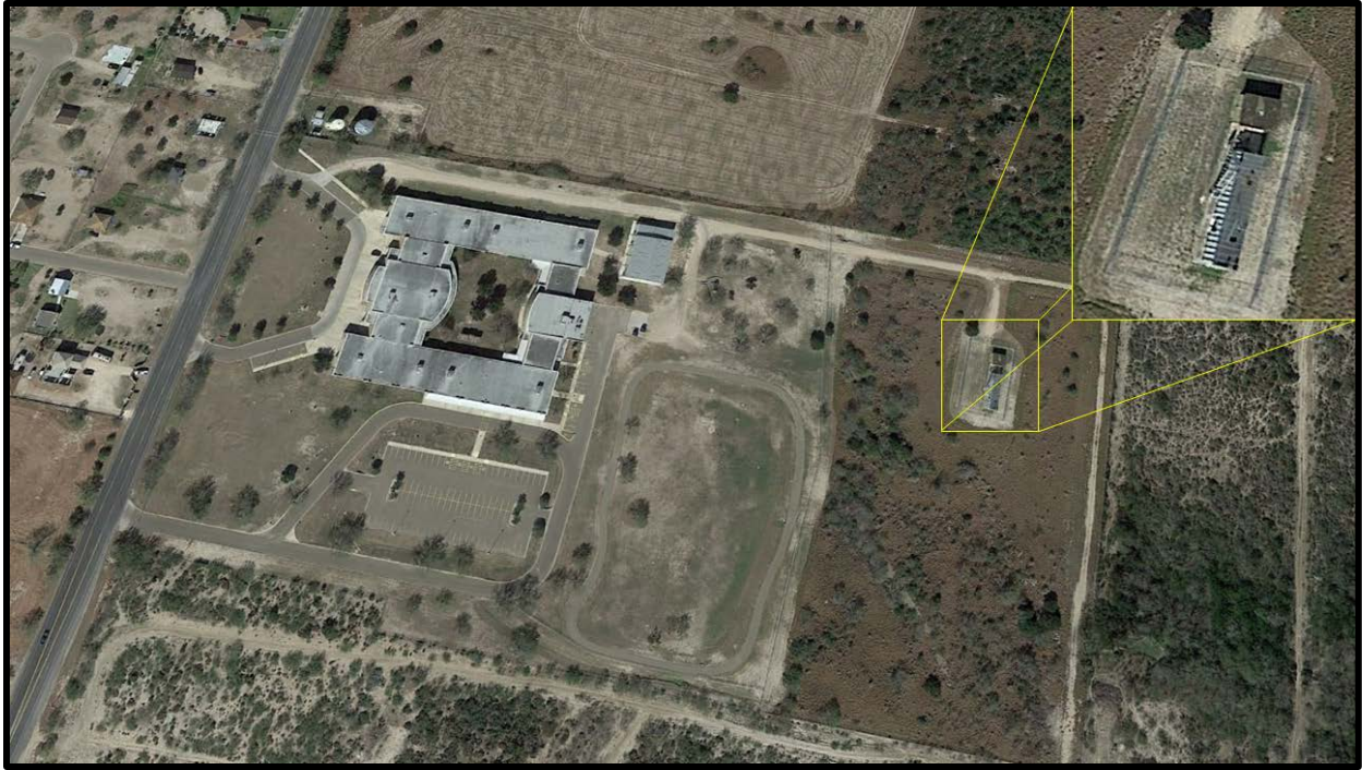
Figure 1-28. La Joya Independent School District's Wastewater Treatment Facility.
