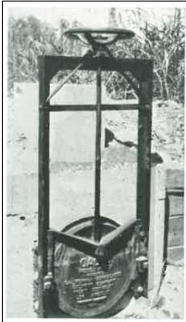
Figure 1. 20" Calco Slide Headgate (Fresno Irrigation District, 1928).
