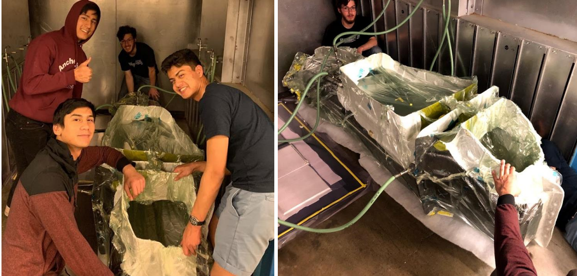
Figure 167. The bag was routed through the rear access hole (left) and had plenty of excess material to remove internal bridging (right).
