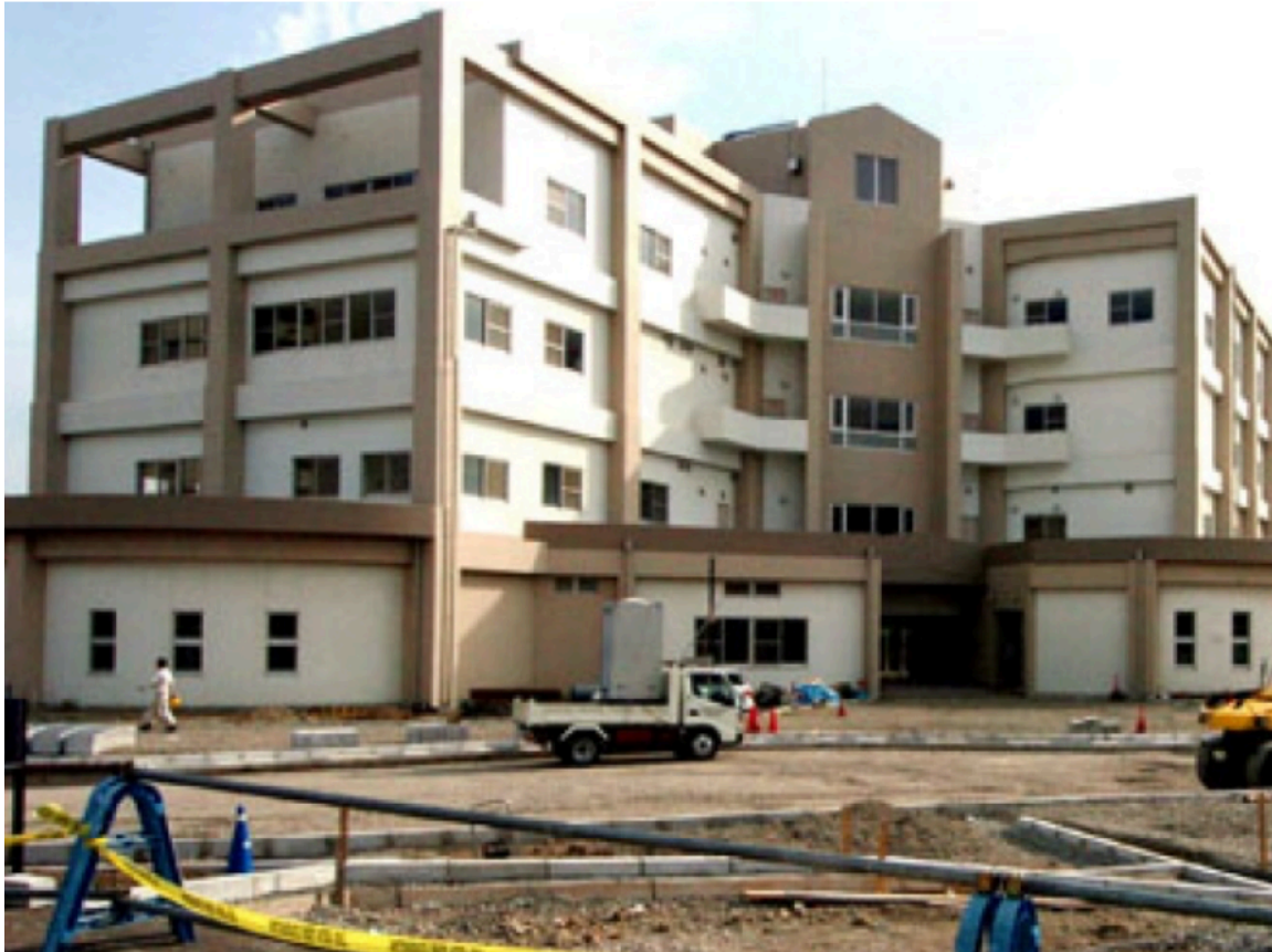
Figure 4: Photograph of subject facility during construction
