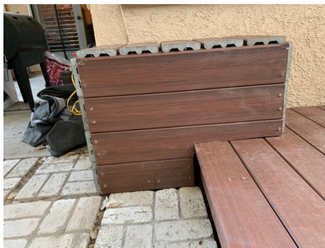
Finished Water Line Housing Unit
