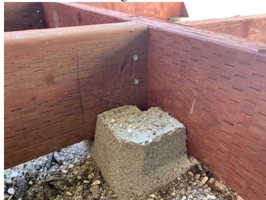
Connection at Concrete Deck Block
