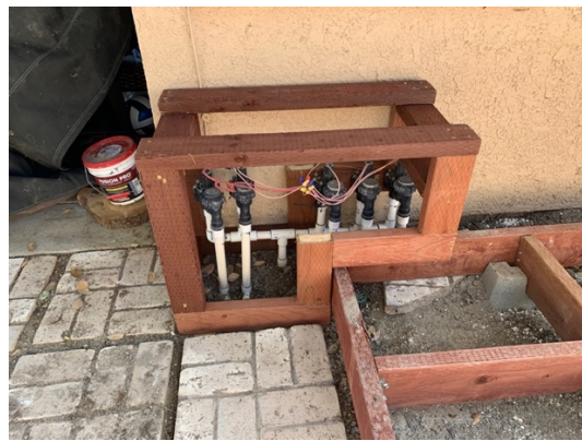
Framing Removable Housing Structure
