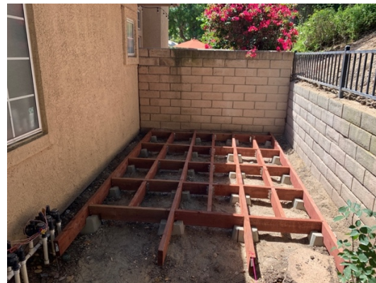
Connection at Concrete Deck Block
