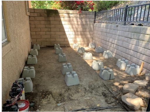
Laying Concrete Decking Blocks
