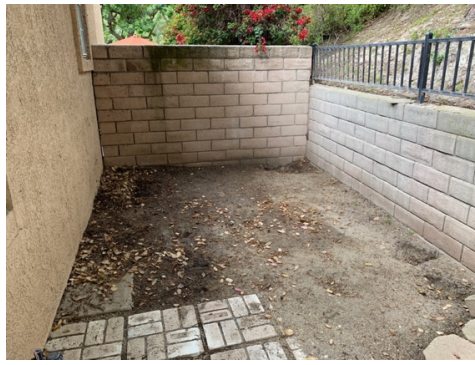
Area Prior to Construction
