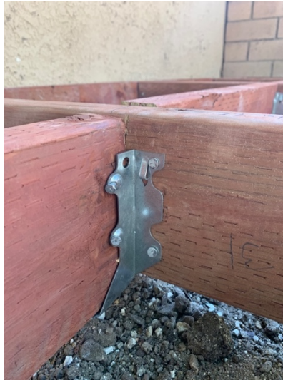
Joist Hanger Connection
