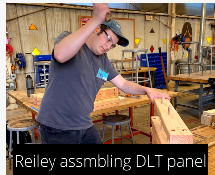
DLT panel in construction
