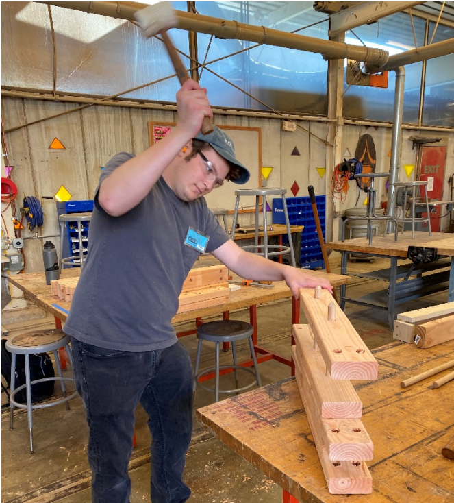
Figure 10: Assembling Individual DLT Panels
