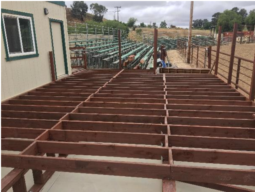
Figure D – Joists run over pony walls
