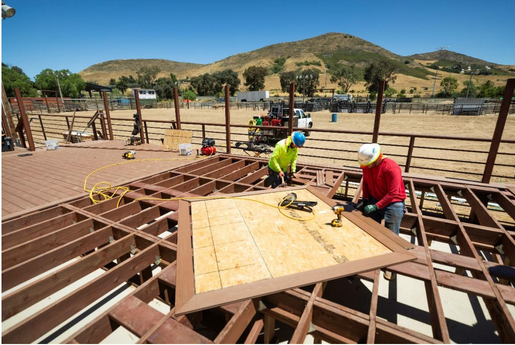
Figure E – Laying out new diamond pattern (courtesy Joe Johnston)
