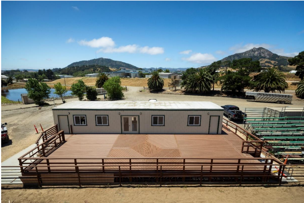
Figure G – Completed deck picture (courtesy Joe Johnston)
