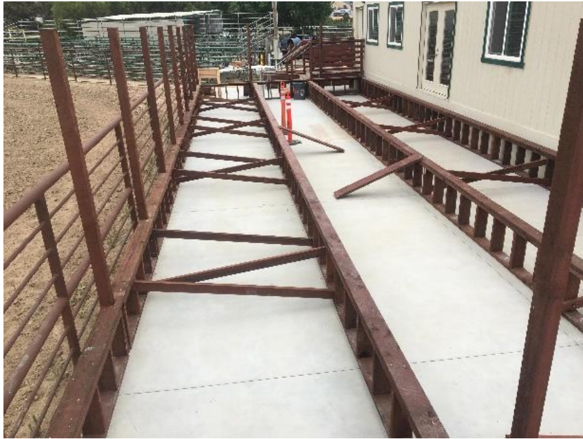
Figure C – Pony walls built with cross bracing installed
