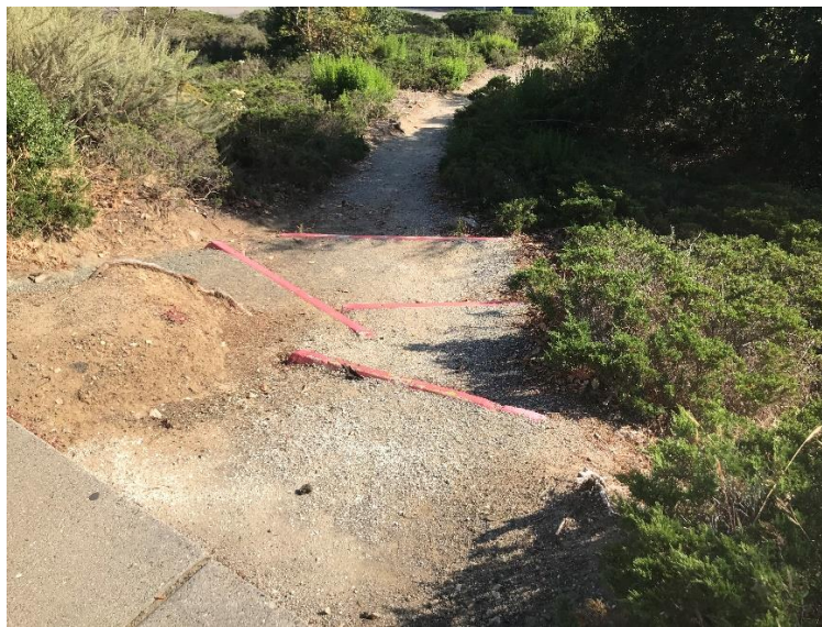
Figure 3. Temporary stairs (Top view)
