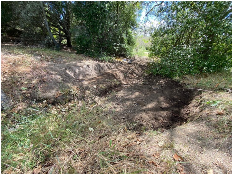
Figure 10 - Site After Earthwork (looking out)
