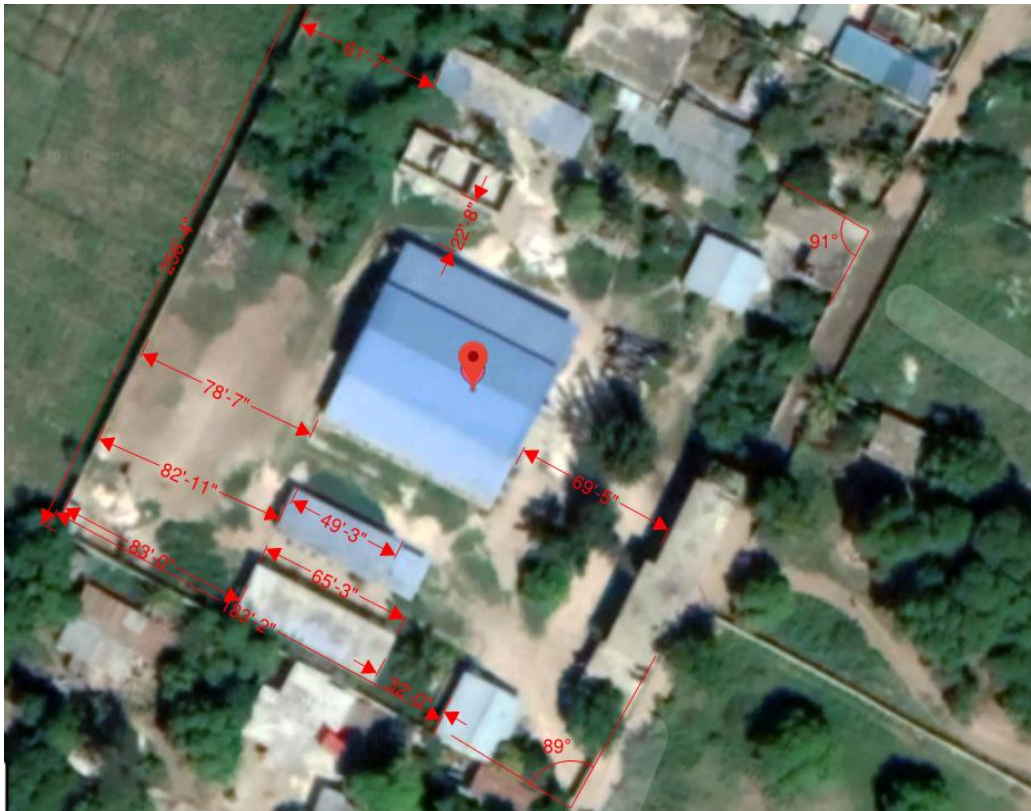
Figure 4. Good Rest Orphanage with angle measurements.
