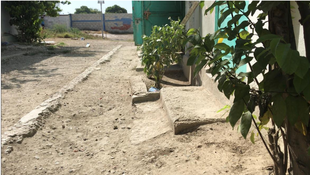
Figure 1. The existing site conditions at Good Rest
