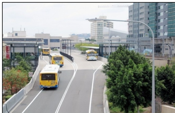
Figure 2-7: Segregated busway (base: http://juts.janes.com )
