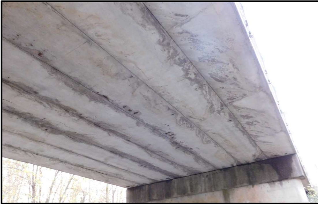
Figure 4.33 Middle span of Main Street Bridge
