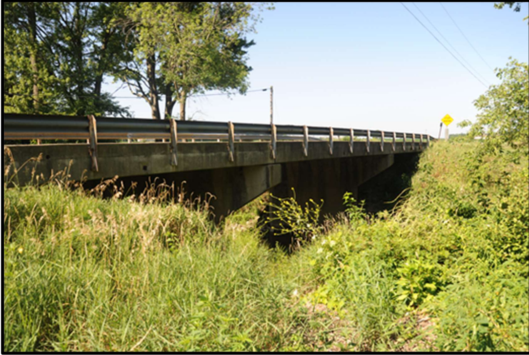
Figure 4.8 Rock creek bridge.
