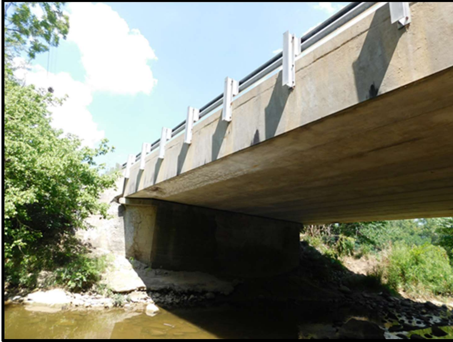
Figure 4.13 Clear creek bridge.
