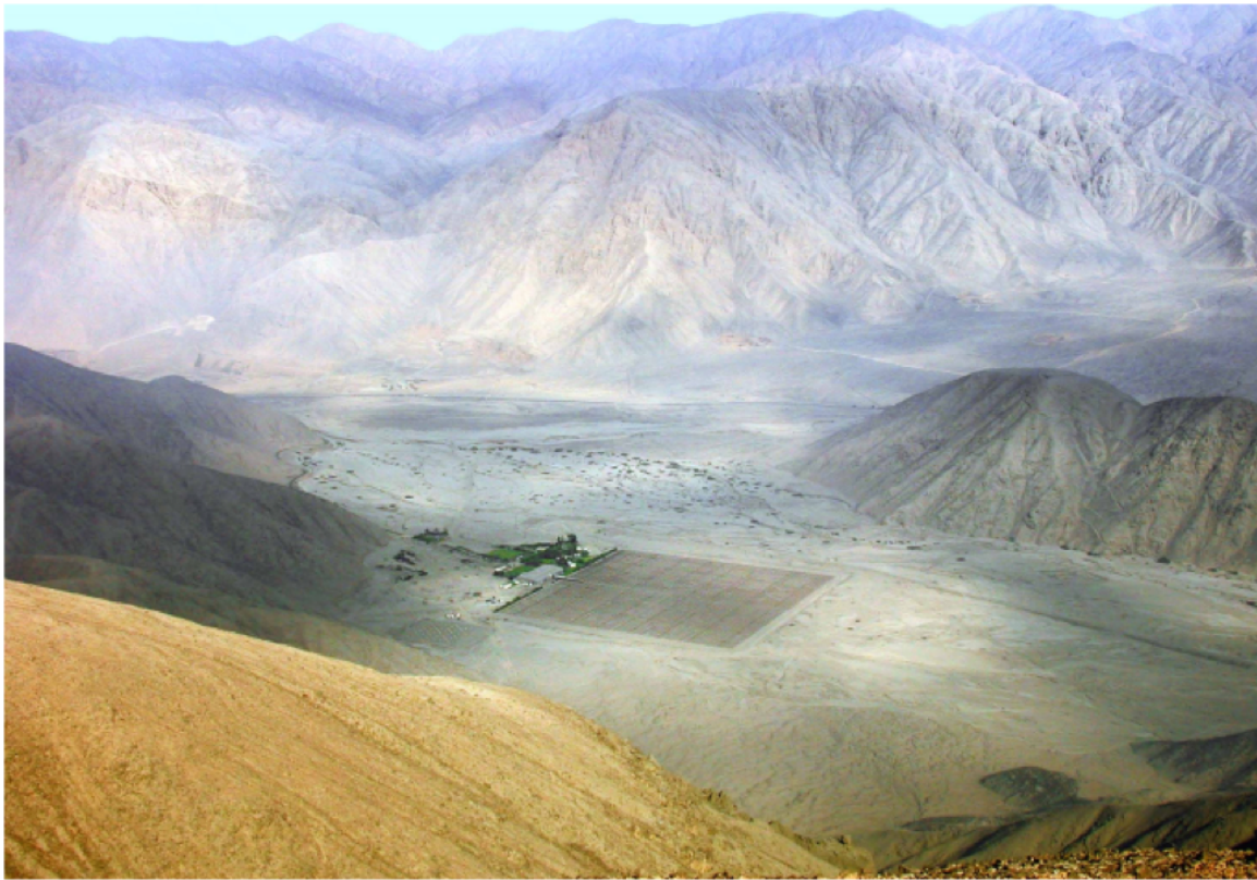
Figure. 3.8: View of the Jicamarca Radio Observatory. The mountains around Jicamarca protect it from electromagnetic interference (Picture taken near the Fabry-Perot Interferometer location. Courtesy of Oscar Veliz).
