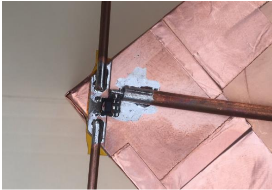
Figure 2.7: Close up of Balun Connection
