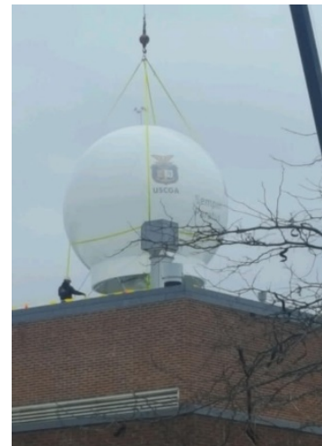
Fig. 1. An MC3 ground station, consisting of a radome housing a 9-meter long antenna, was placed on the roof of the Science building at CGA for use in the Polar Scout mission, and beyond.
