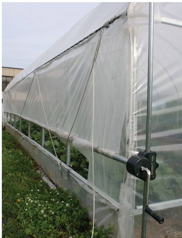
Figure 19. Roll-up window vent with “W” rope lacing to prevent blow-out of sidewalls in high winds.
