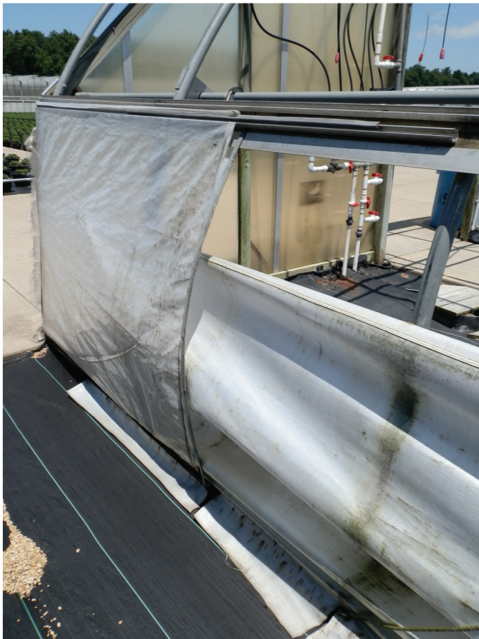
Figure 7. Drop down sidewalls ( above and adjacent ) are preferred since ventilation occurs above the plants rather than near the ground, which can slow plant growth and increase the potential for cold injury.
