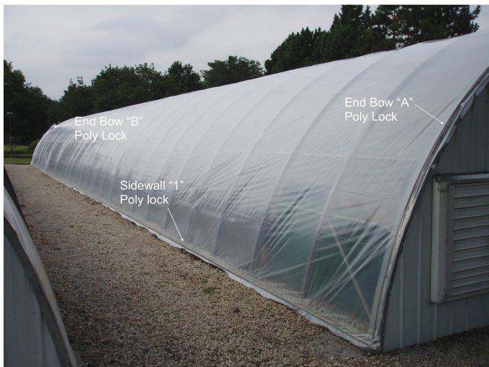
Figure 18. Locations of end bow and sidewall poly-locks.
