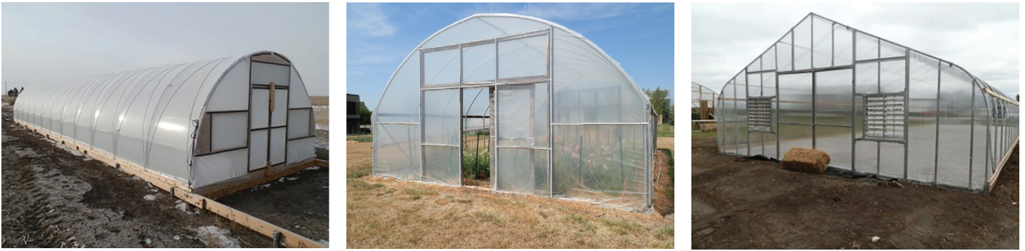
Figure 2. Common high tunnel profile designs include the hoop ( left ), raised hoop ( center ), and peaked hoop ( right ).
