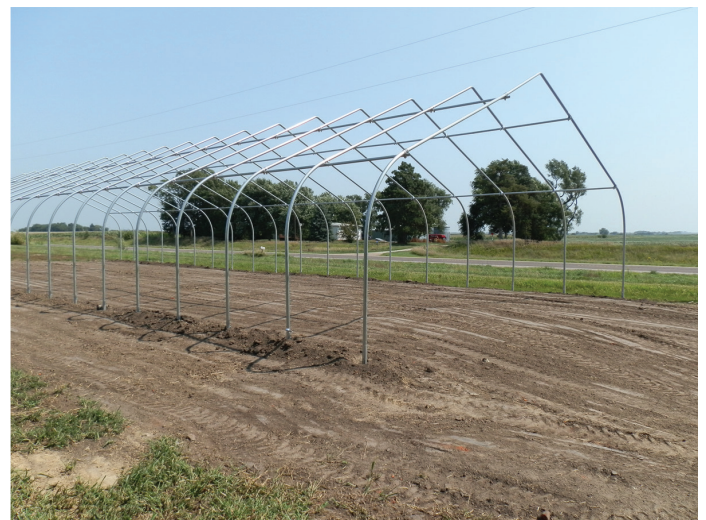
Figure 9. Creating a level site through cut and fill excavation will result in compacted soils that are unlikely to be suitable for in-ground plant production.
