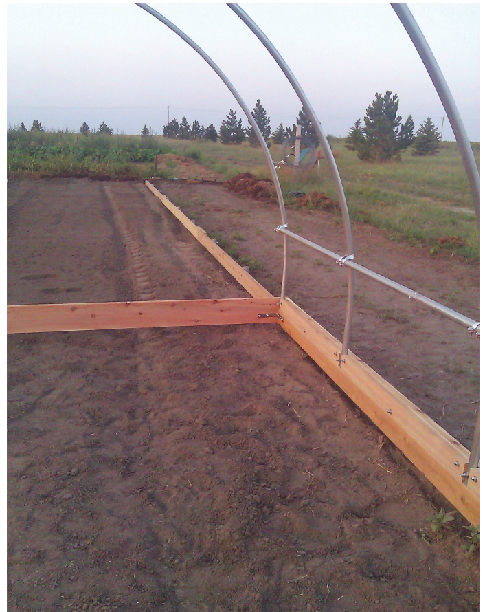
Figure 16. Wood baseboards have been installed in a new high tunnel.
