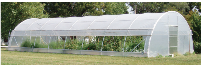
Figure 5. Roll-up sidewall components provide options for improved interior temperature management. Note overlapping wall blanks at both ends of the roll-up wall to prevent cold air infiltration.
