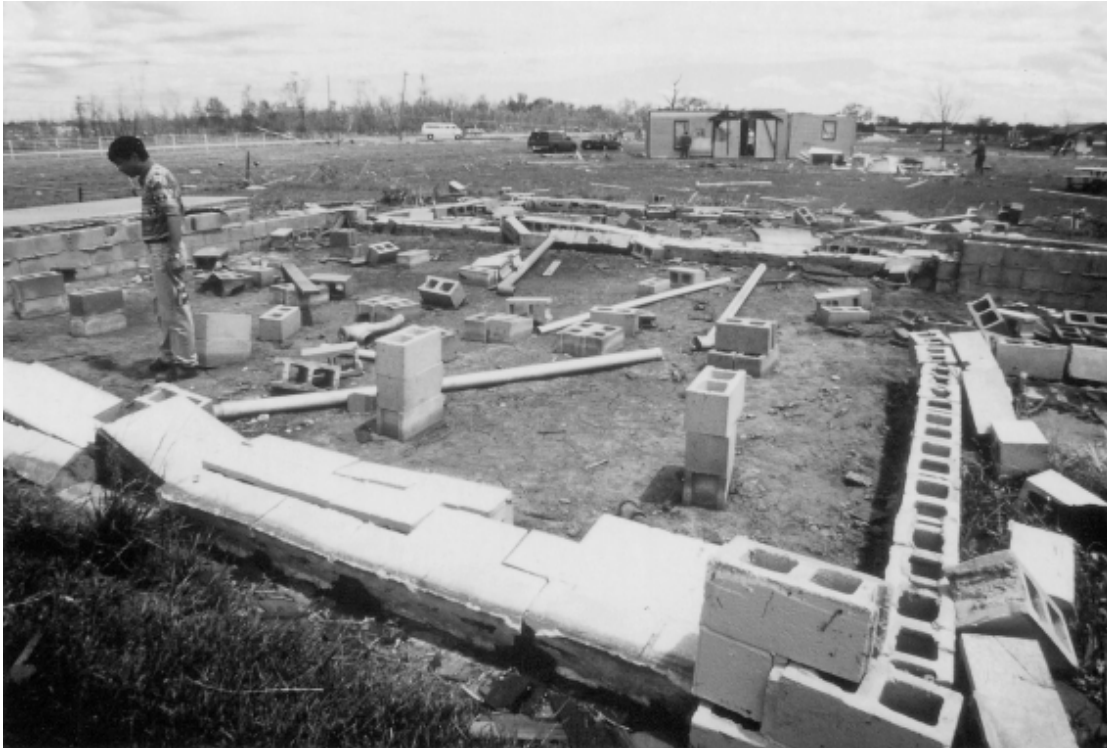
Figure 5.21, House shifted off foundation 90 m in Moore, OK after 1999 tornado (Marshall, 2002).
