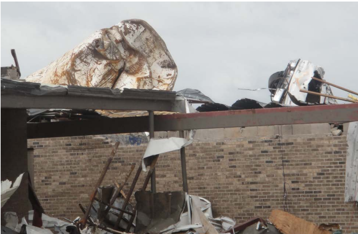
Figure 6.30, Oilfield Tank on Briarwood Elementary School Roof
