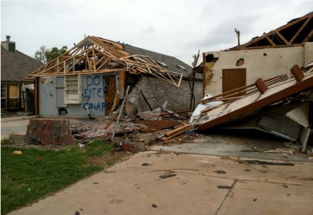
Figure 5.2, Garage removed from house on left with protruding garage.
