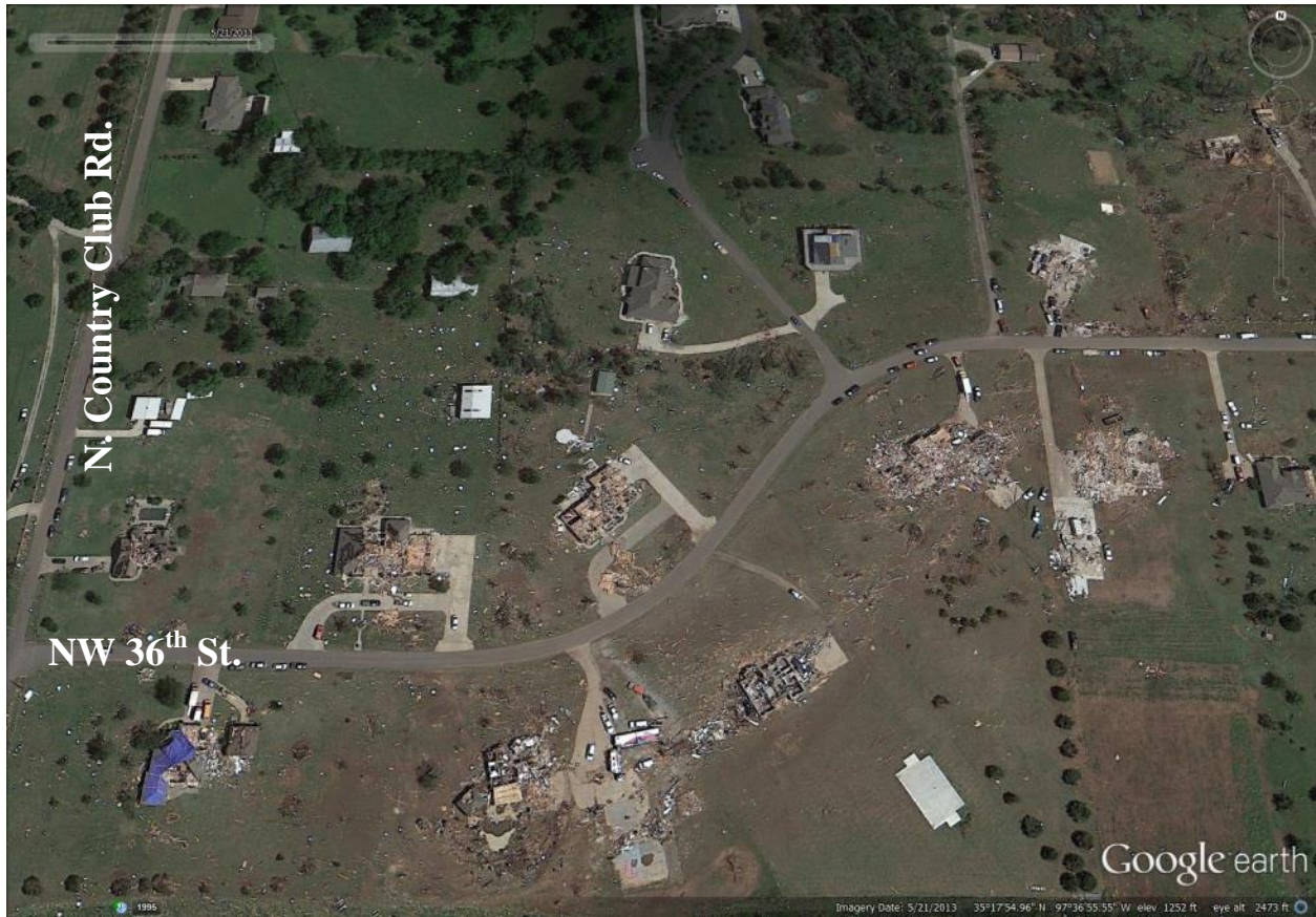
Figure 6.3, Damage in Newcastle neighborhood (NW 36th).
