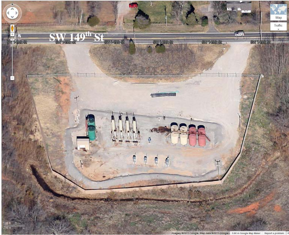
Figure 6.27, Tank Farm Undamaged Condition.
