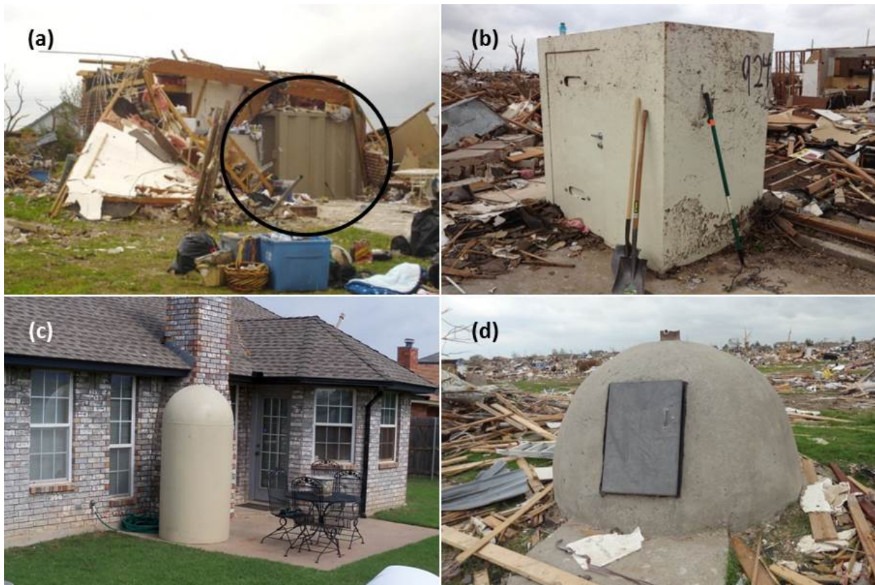
Figure 4.8, Residential shelter images; (a) and (b) steel storm shelters bolted to the garage slab; (c) cylindrical steel exterior storm shelter; and; (d) homemade concrete dome refuge.
