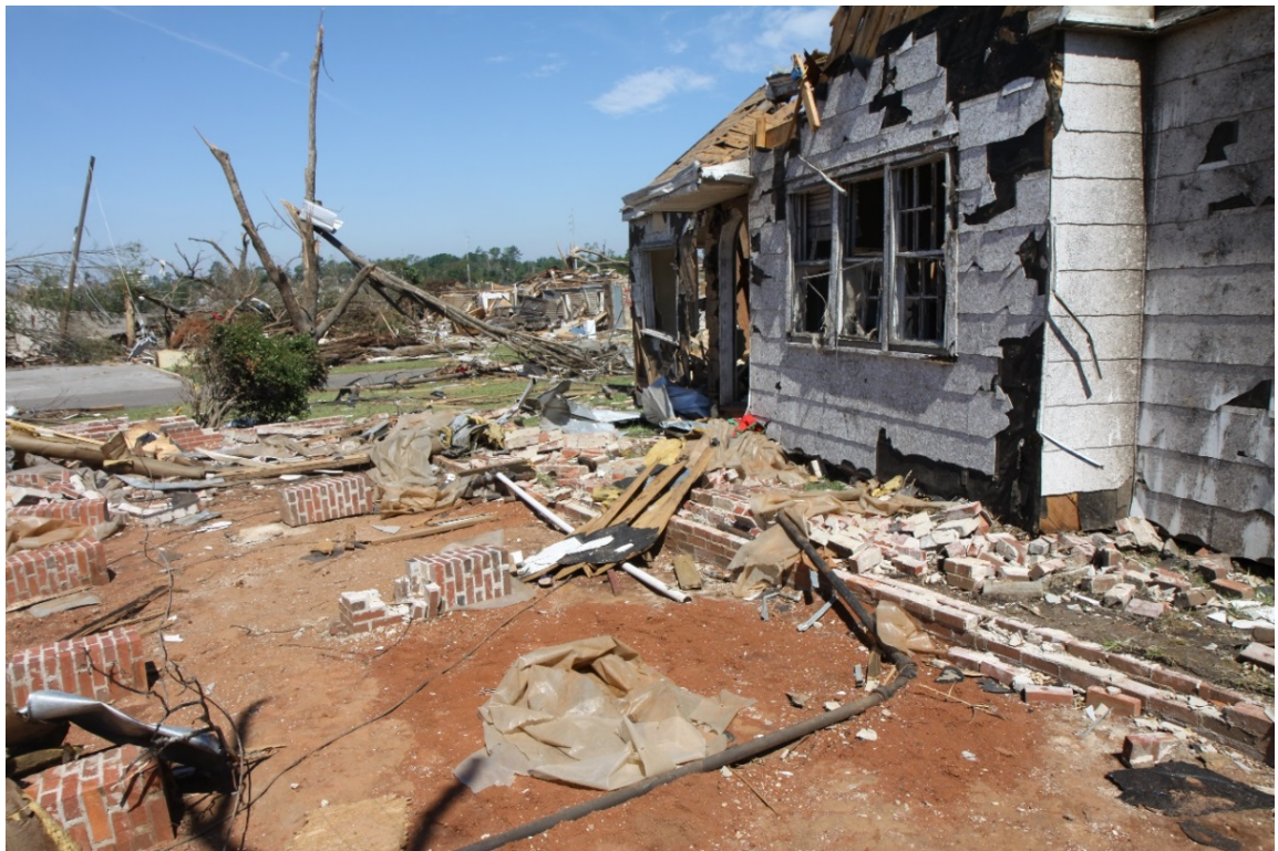
Figure 5.20, House shifted off of crawlspace foundation in Tuscaloosa, AL after 2011 Tornado.
