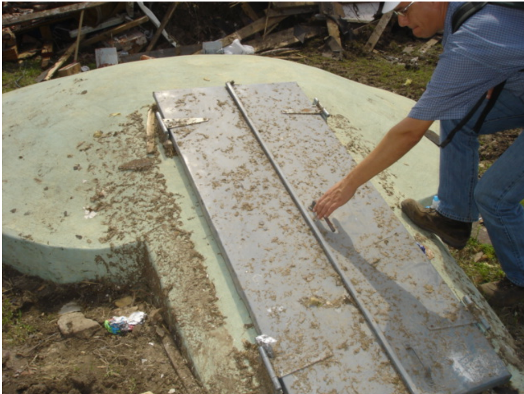
Figure 4.13, This shelter was one of the older observed shelters in the area.
