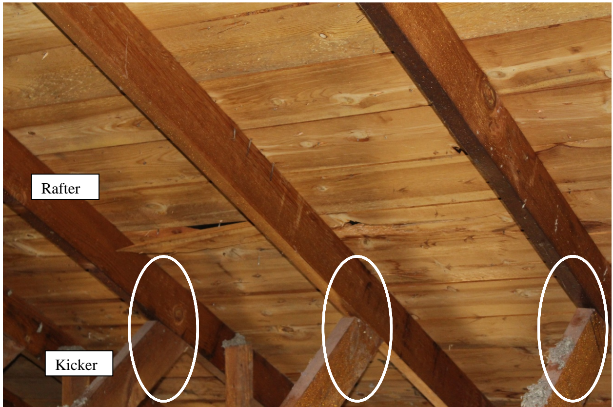
Figure 5.28, Typical Roof Truss Connections
