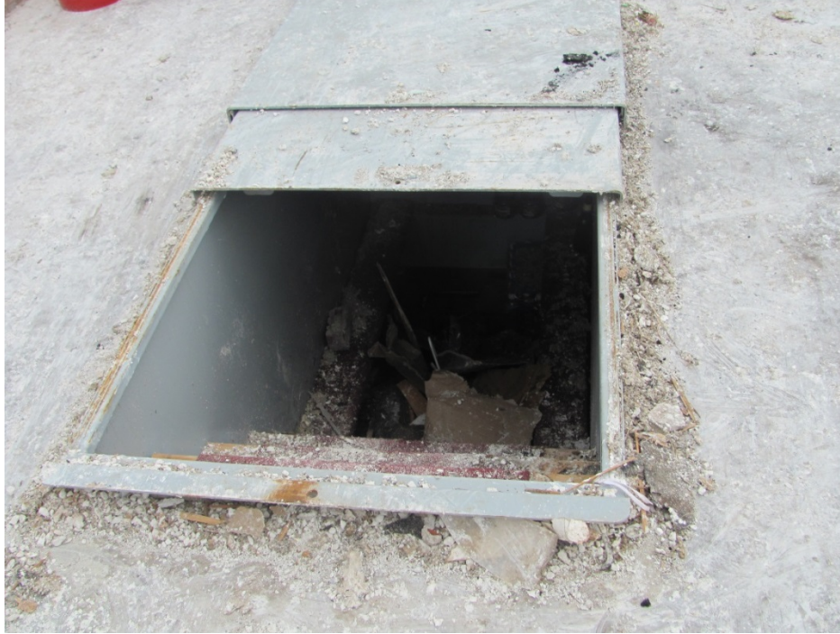
Figure 4.3, Example of a garage slab storm shelter.
