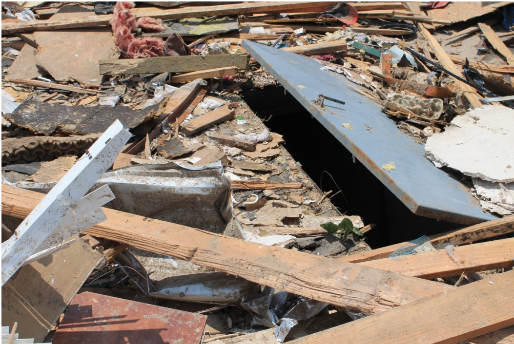
Figure 4.4, Debris blocked storm shelter after an attached garage failed.
