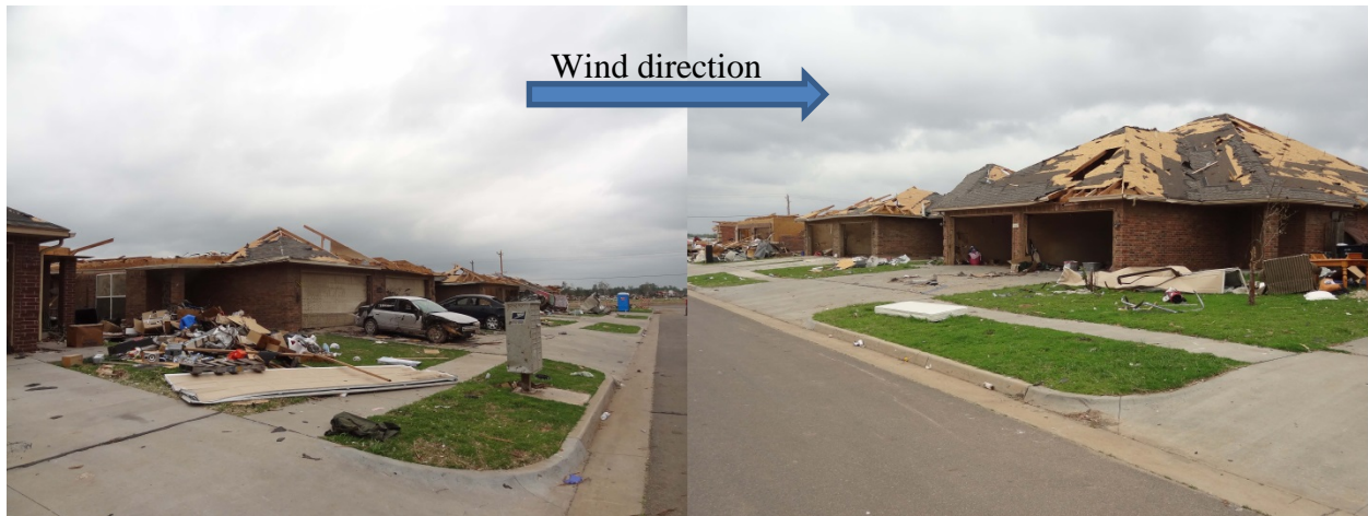
Figure 7.4, Failure of roofs and garage doors on (a) west side and (b) east side of Kyle Dr.
