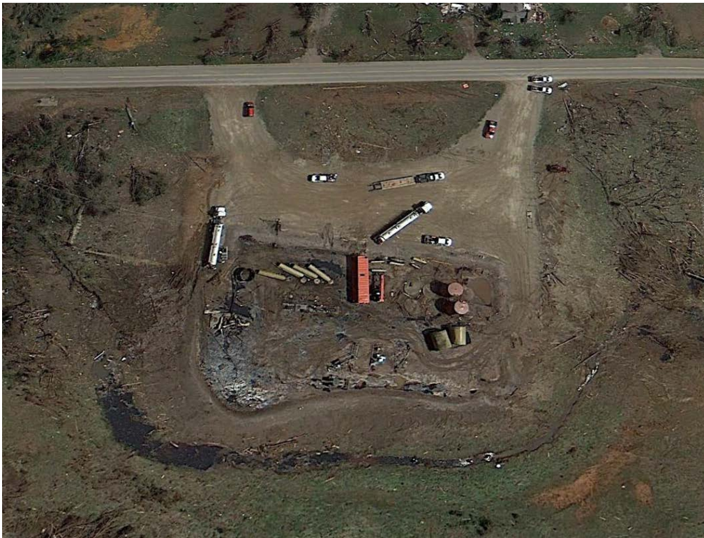
Figure 6.28, Damaged Tank Farm
