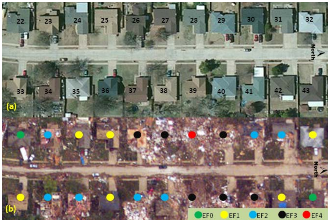
Figure 2.10, Aerial images and EF rates of the area #2: (a) pre-tornado image and building IDs; (b) post-tornado image and EF rates.
