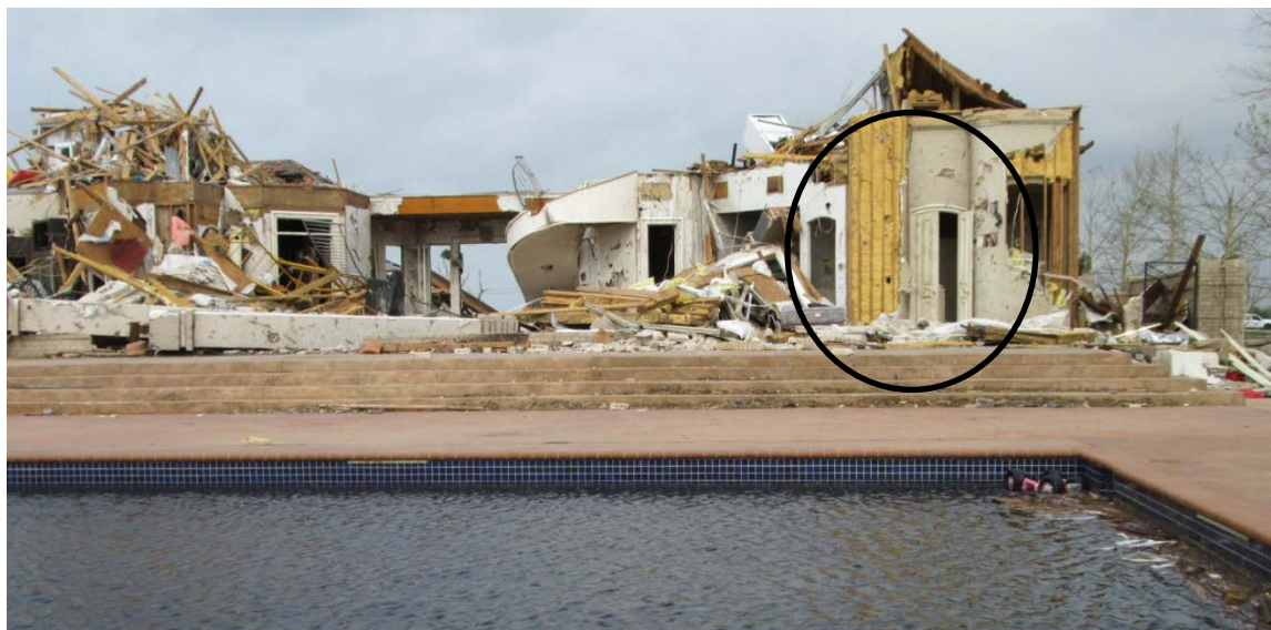
Figure 4.7, FEMA designed CMU safe room found near SW 149th St and S. May Ave. The safe room is centrally located among the remaining rooms and is indicated with the black circle.
