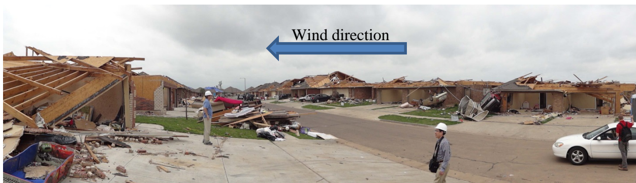
Figure 7.3, Damage pattern on Kyle Dr., Moore, Oklahoma (Camera pointed to the south).
