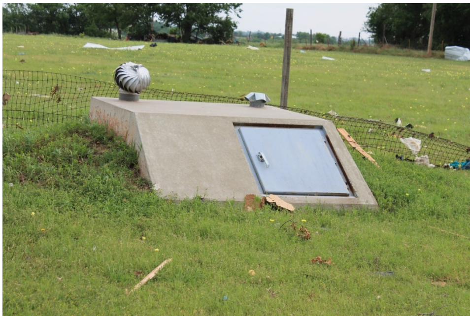
Figure 4.2, Example of a prefabricated concrete storm shelter.
