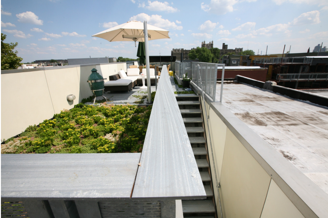
Figure 8: Jackhammer, communal space
