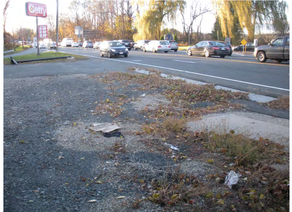
Figure 3.12 shows exposed soil that is not native to the area
