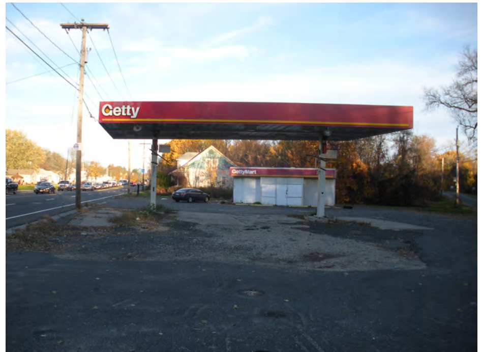
Figure 3.19 shows the area where the underground fuel storage tanks were located
