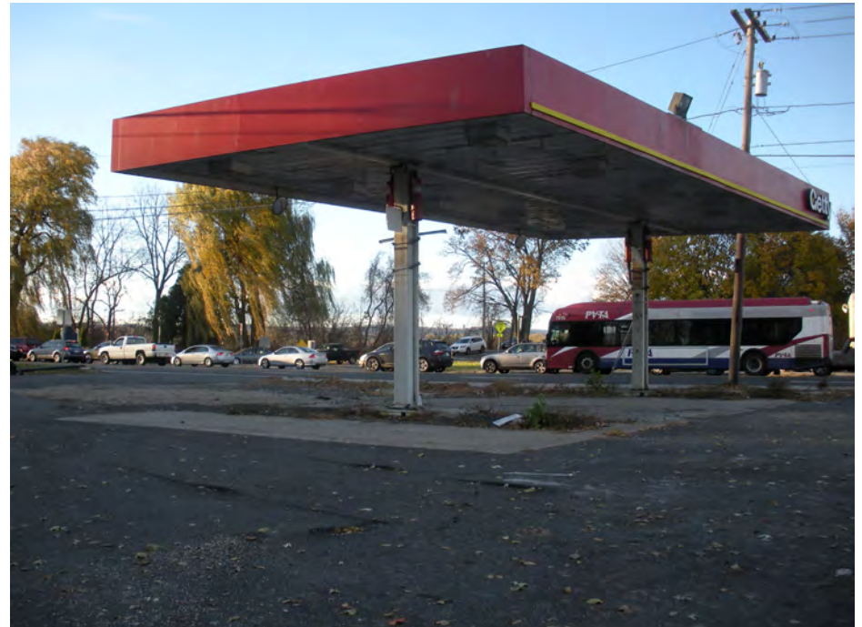
Figure 3.18 shows existing overhead canopy
