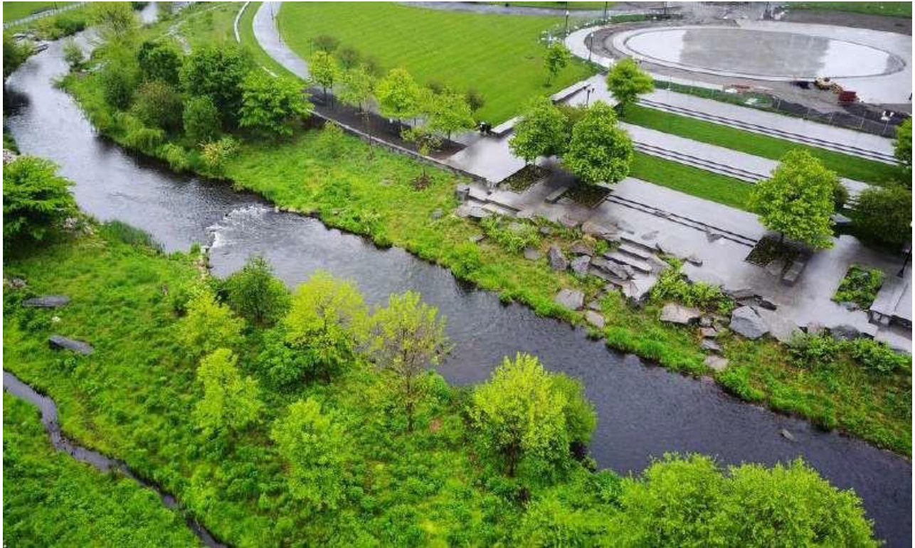
Fig. 8: The newly naturalized banks of the Mill River designed with access points down to the water's edge. (Courtesy of OLIN 2014)
