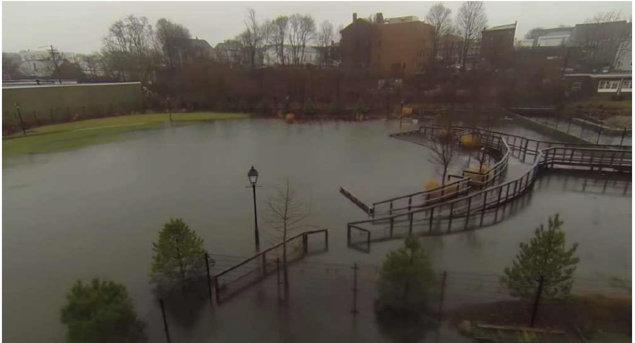
Fig. 28: Veteran Memorial Park during a flash flood in 2016 acts as a retention pond for stormwater runoff. (Courtesy of Salem News)
