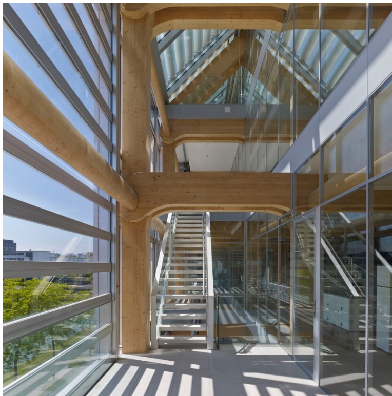
Figure 12. All-timber structural system of the Tamedia Office Building (Shigeru Ban Architects; Zurich, Switzerland; 2013). Photo by Didier Boy de la Tour.
