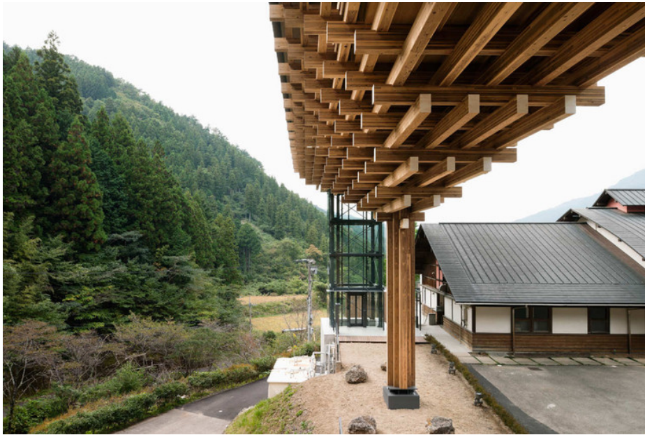
Figure 11. Joinery detail at the Yusuvara Wooden Bridge Museum (Kengo Kuma & Associates; Yusuvara, Japan; 2011). Photo by Takumi Ota.
