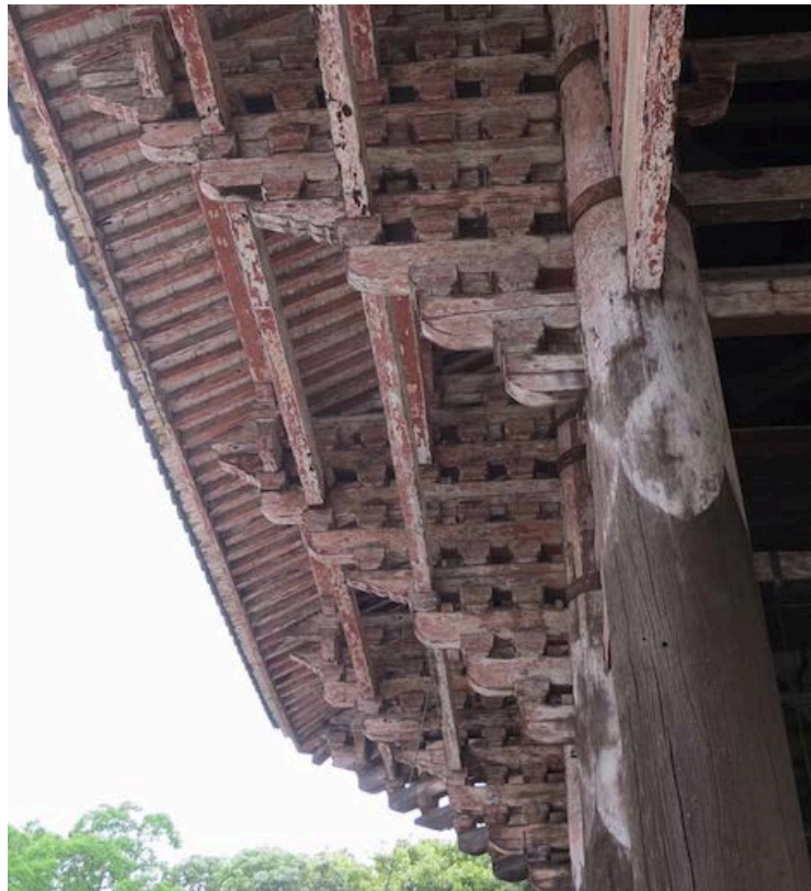
Figure 6. Bracket set joinery at Nandaimon, or the Great South Gate (Nara, Japan; 12 th century) of Todai-ji. Photo by Deanna MacDonald.
