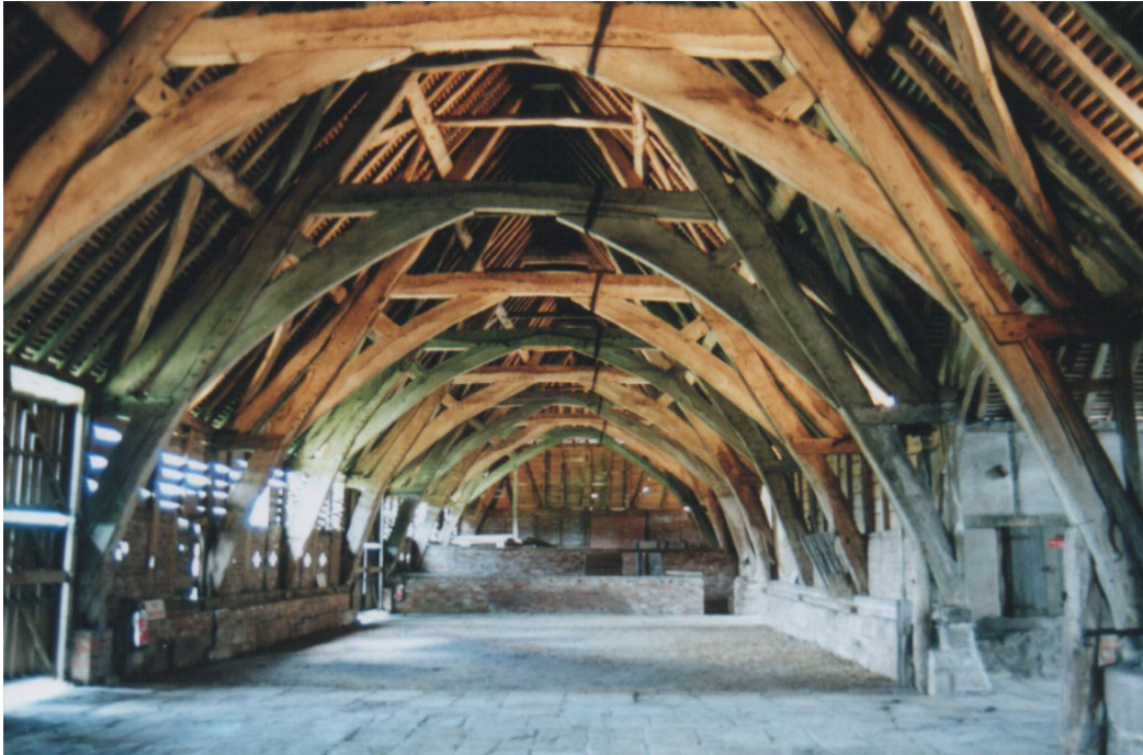
Figure 8. Cruck framing, an English carpentry technique. Leigh Court Barn is the largest cruck framed structure in Britain (Worcester, England; 1325). Photo by Simon Webb.
