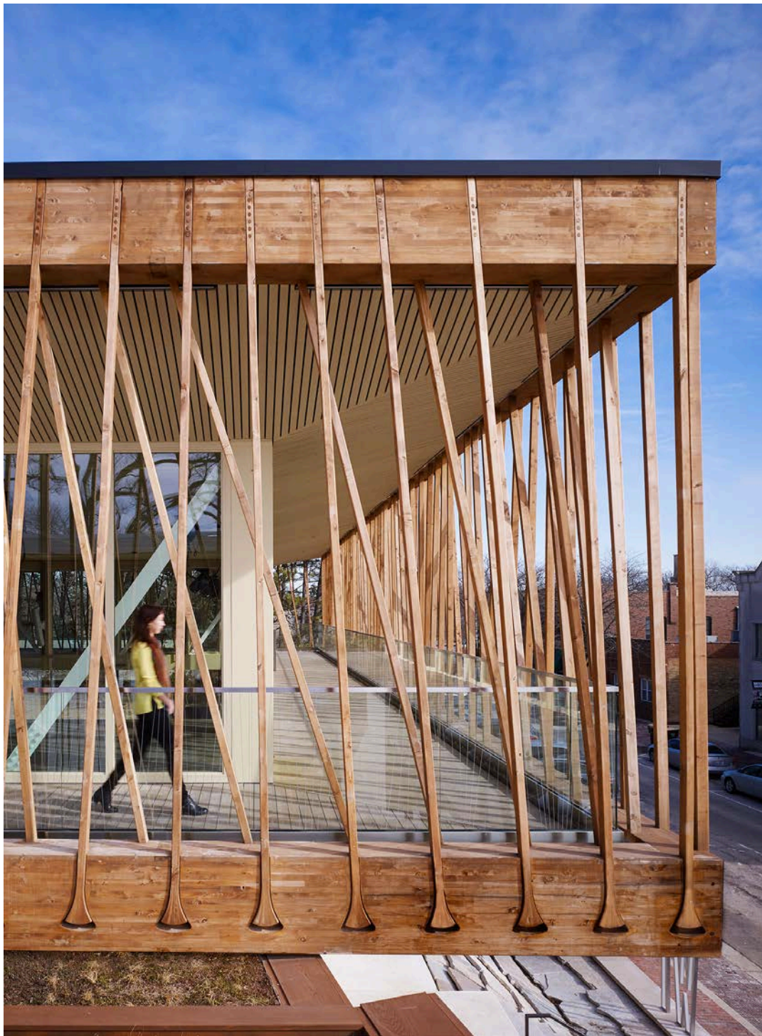
Figure 13. "Cat's paw" timber tension joinery detail at the Writers Theatre (Studio Gang; Glencoe, IL, USA; 2016). Photo by Steve Hall © Hedrich Blessing.
