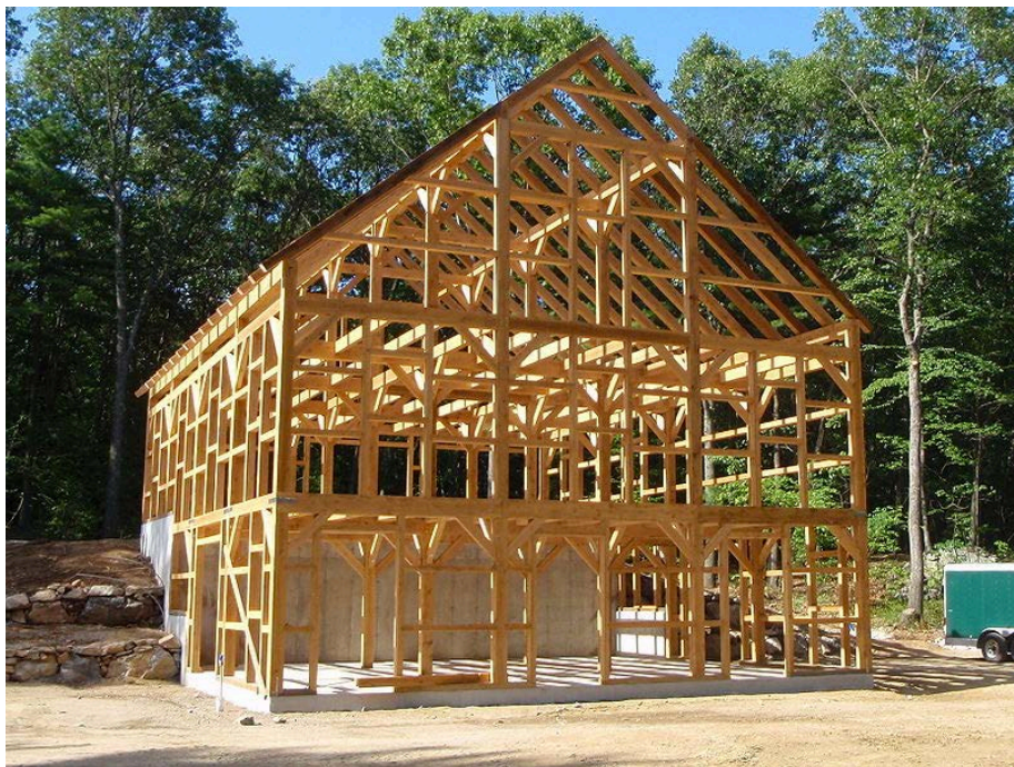
Figure 9. A modern example of North American timber framing tradition. Photo by Vermont Timber Works Inc.
