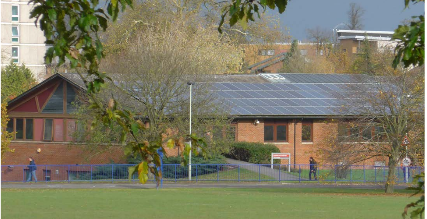
Figure 5.1 Solar PV panels on the Estates & Facilities Building, University of Reading
