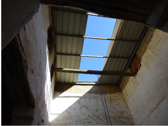
Figure 4: Partially Covered Courtyard
