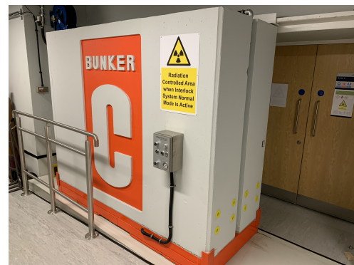
Figure 2. The floating concrete door and entrance to the shielded bunker C.
