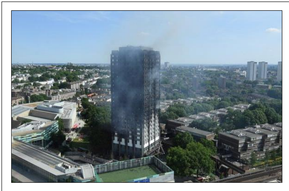
Figure 2-2: Grenfell Tower in west London after the fire [51].
