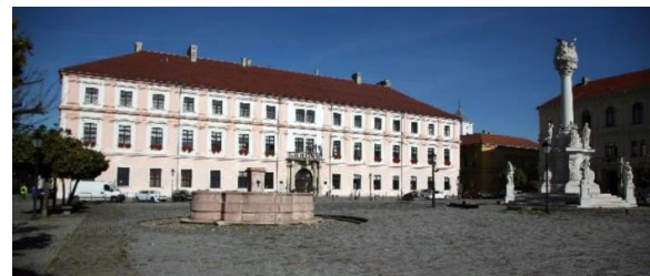
Figure 3: The Palace of the Slavonian General Command in Osijek in northern Croatia. (Stober et al. , 2018)
