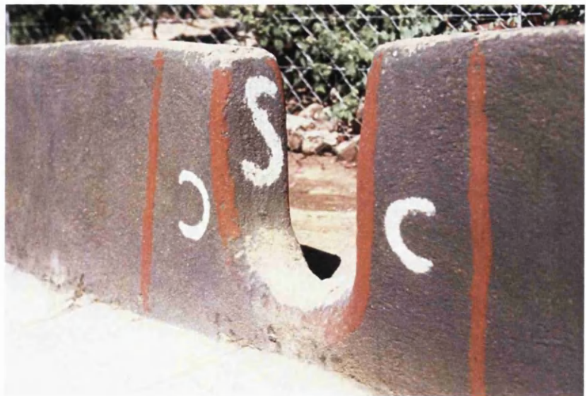
Figures 1.29, 1.30 and 1.31 Repeated symbols used at the corners and entrances to the lolwapa. Oodi, 1996.
