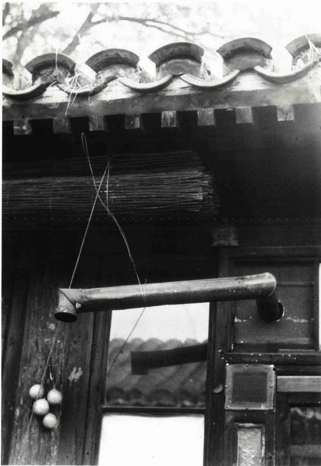
Solutions to Beijing's extreme climate: stove pipe and bamboo sun-blinds
