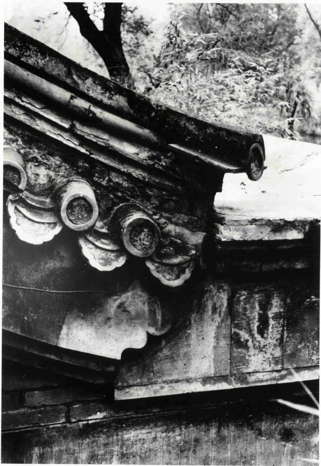
The Z house: roof detail
