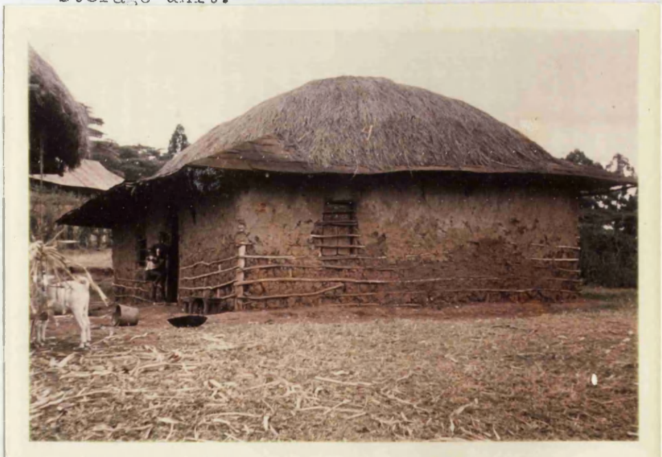
6. Similar local housing in Gakarara. The roof is covered with both old tin and grass; the mud and wattle construction is clearly shown.
