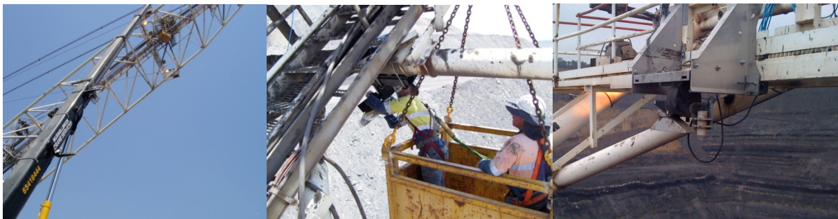
Figure 2 - Sensor Package Location, Left and centre: showing the installation to the first mounting location. Right: showing the second location on landing.
