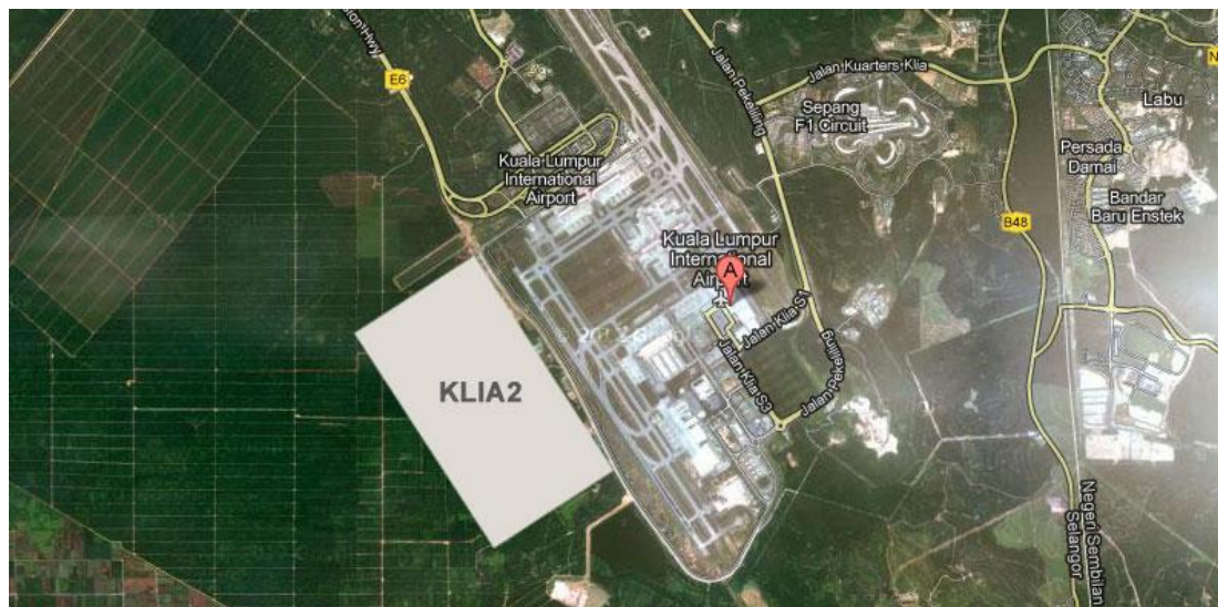
Figure 7 KLIA2 Site Location in Sepang, Malaysia (Source:www.klia2.info)
