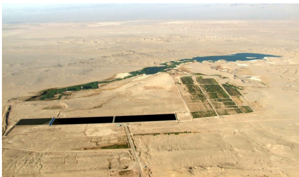
Figure 1. Overview of treatment plant
