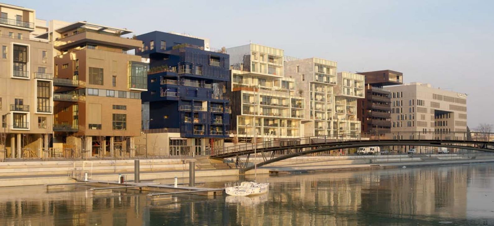
Massimiliano Fuksas, Vincenzo Amantea, Clément Vergély e H.T.V.S Architecture, Buildings in Place Nautique
