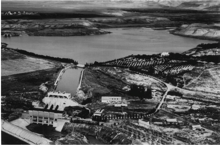
Figure 3.6: The Rutenberg-Abdallah lake around 1930, on the left the canal leading to the turbines and power station. On the right, next to the lake is the white house of Rutenberg. (Courtesy of the Israeli Electric Corporation archives)
