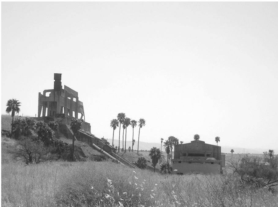
Figure 3.5: A picture of the ruins of the Jordan Power House at Naharayim/Baqora taken from the Jordanian side of the Park. The water entered from the left and flowed through the turbines on the right. A few palm trees from the Tel Or settlement figure in the background. (Photo by Dorien Vanden Boer)
