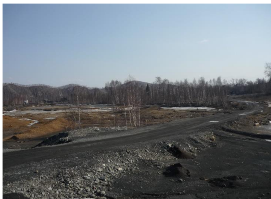
Fig. 7. Using sand for construction of temporary motor roads.
