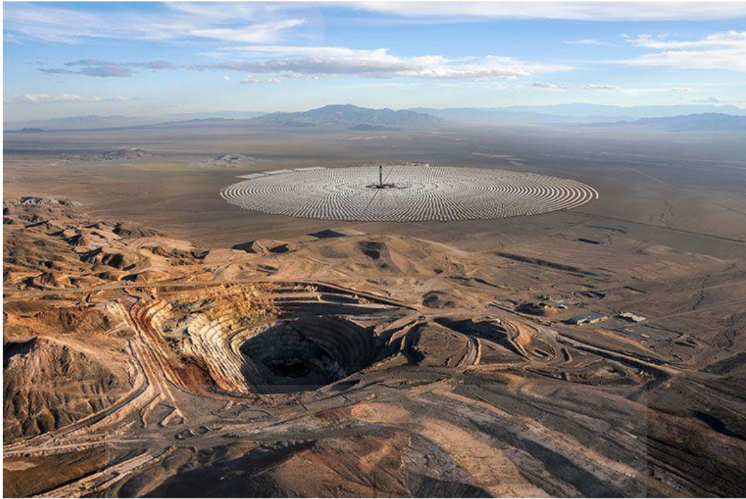
Figure 2.11: The use of CSP with molten salt energy storage to supply power to a mining site (Parrado et al, 2016).
