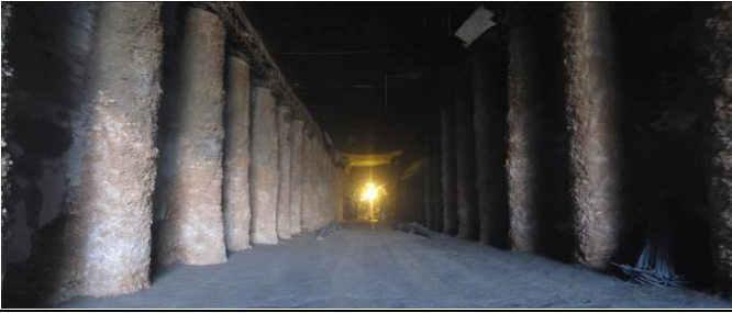
Fig 6 Top/Down method in T4 section
