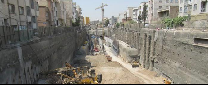
Fig 5 Cut & Cover method in T2 section
