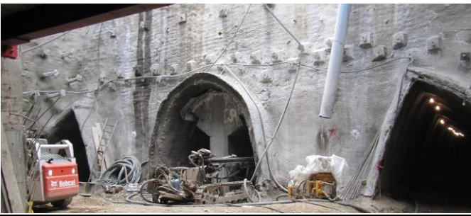
Fig 7 Nailing at TU Portal area
